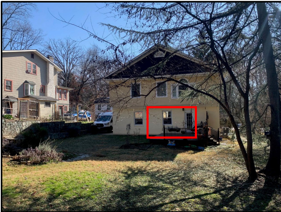
Figure 3: The rear elevation of the existing building. The rectangle indicates the location of the proposed mudroom addition.
