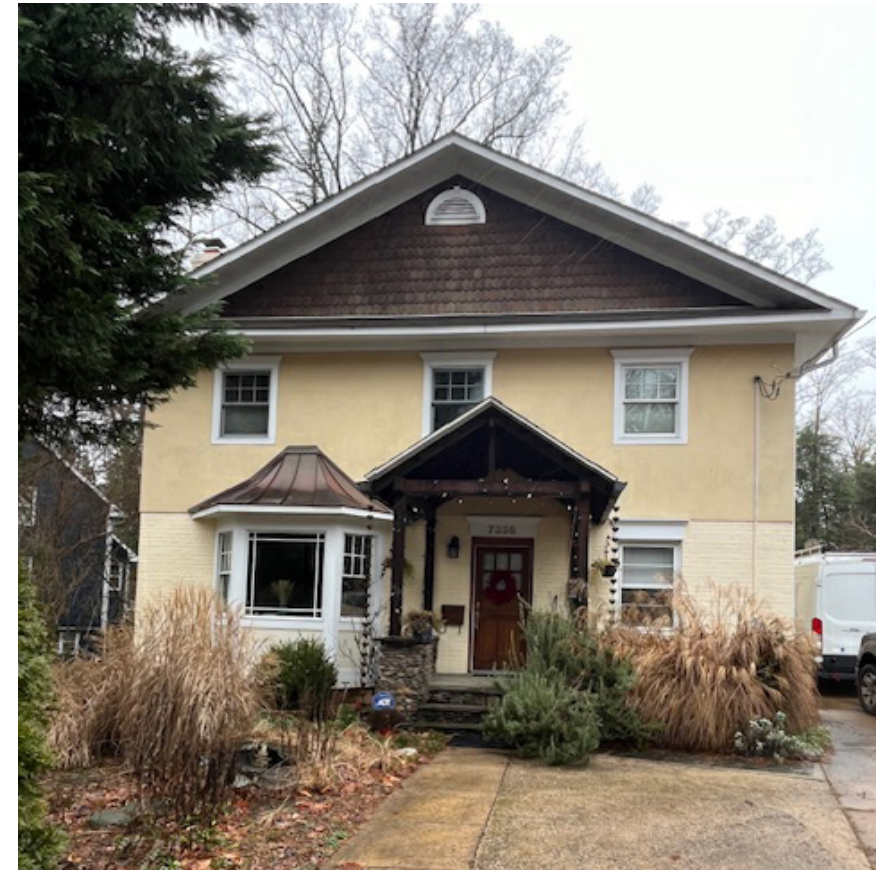
3. NORTH ELEVATION - FRONT OF EXISTING STRUCTURE
