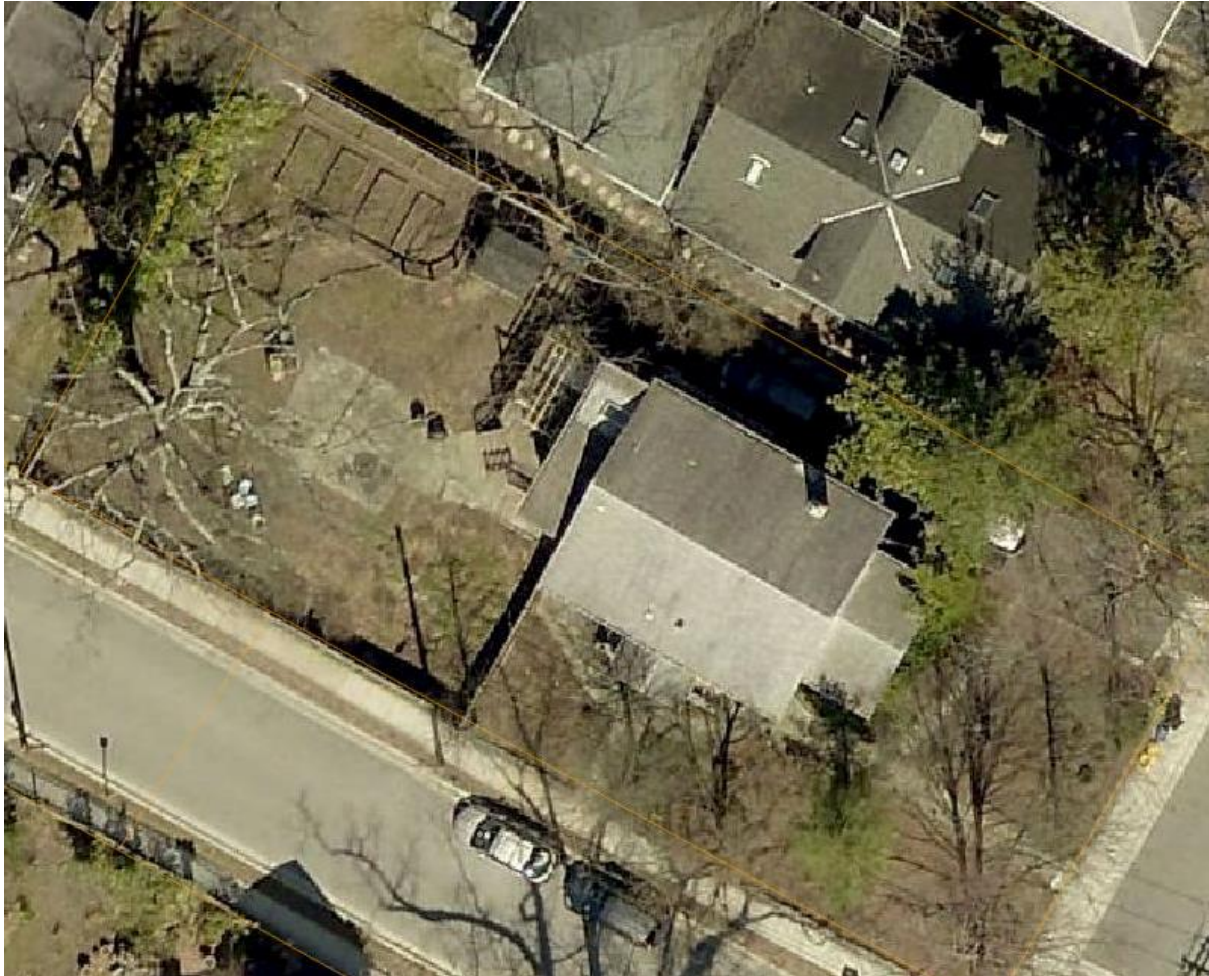
Figure 3: Detail of the subject property. Note the chimney on the north roof slopes and the vents on the south.
