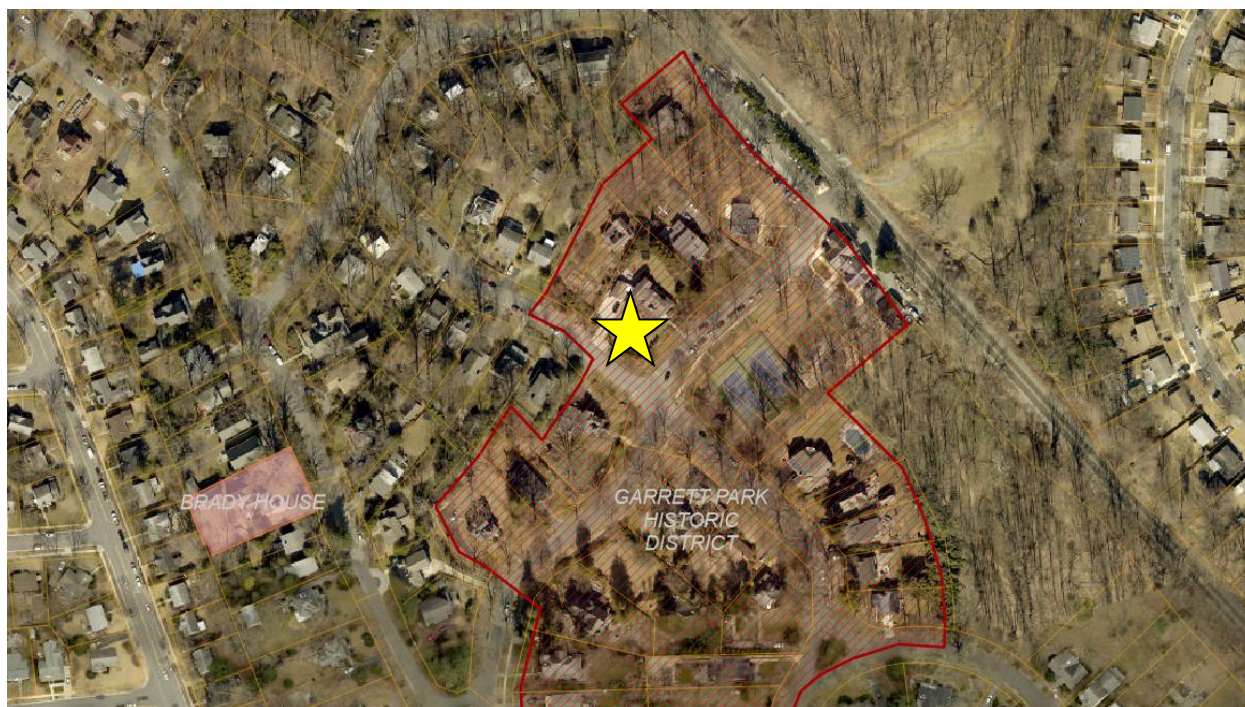
Figure 1: The subject property is located at the intersection of Waverly Ave. and Montrose Ave.
