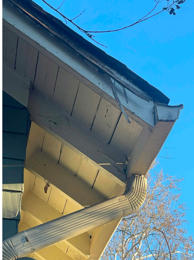
511 Philadelphia Avenue | Sample photos of repairs needed to existing exterior trim
