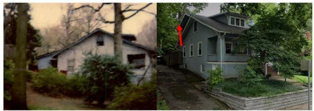
Figure 4: View of the side elevation of 7421 Maple Avenue prior to raising the roof (left) and view of the façade and side elevation after raising the roof (right). The red arrow points to the retention of the original roof form. Sources: Montgomery Planning and Google
