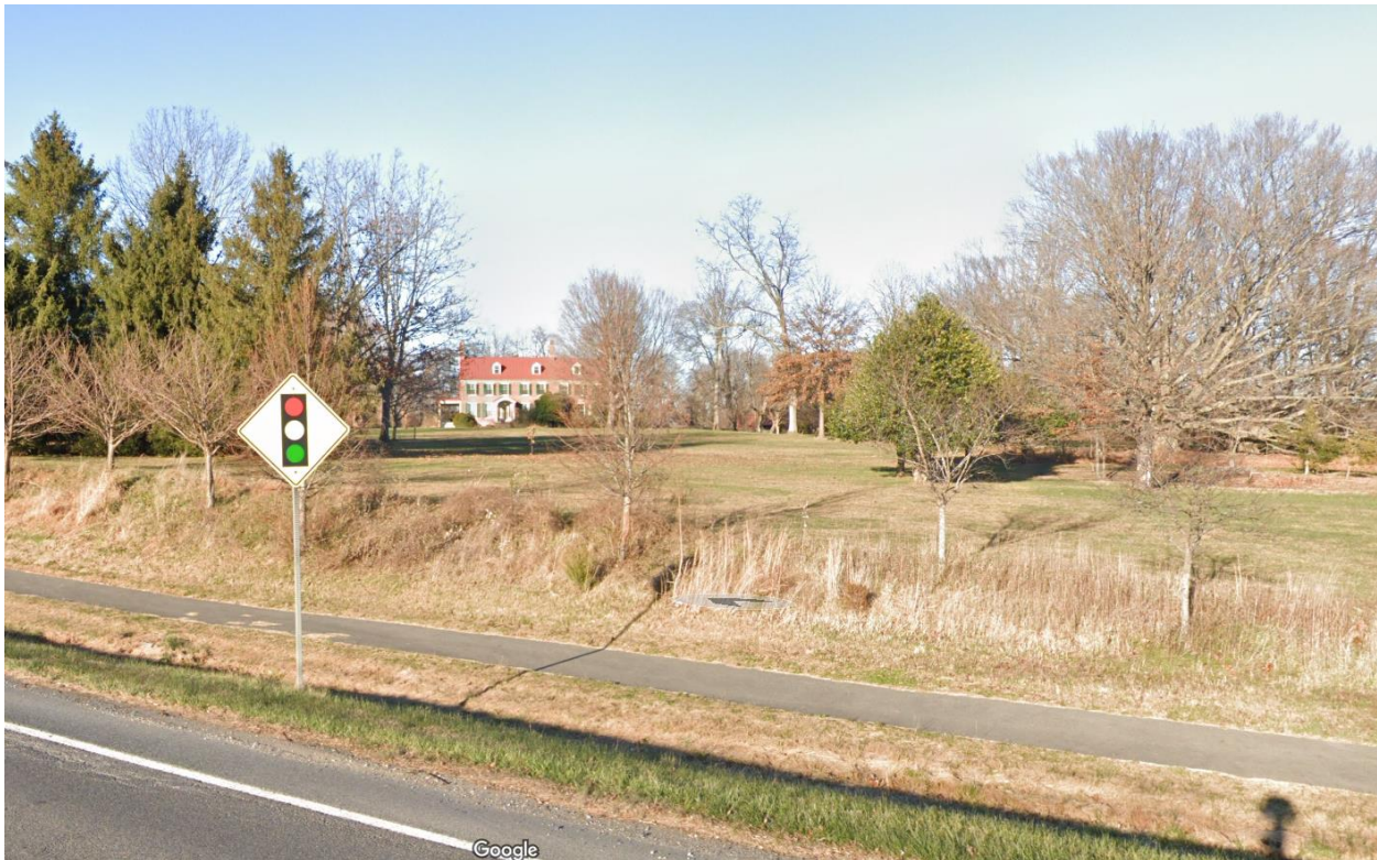
Photo 4: Norwood property, Norwood dwelling, and SUP, looking north from just north of Hennessy Terrace (Google Street View, November 2022)
