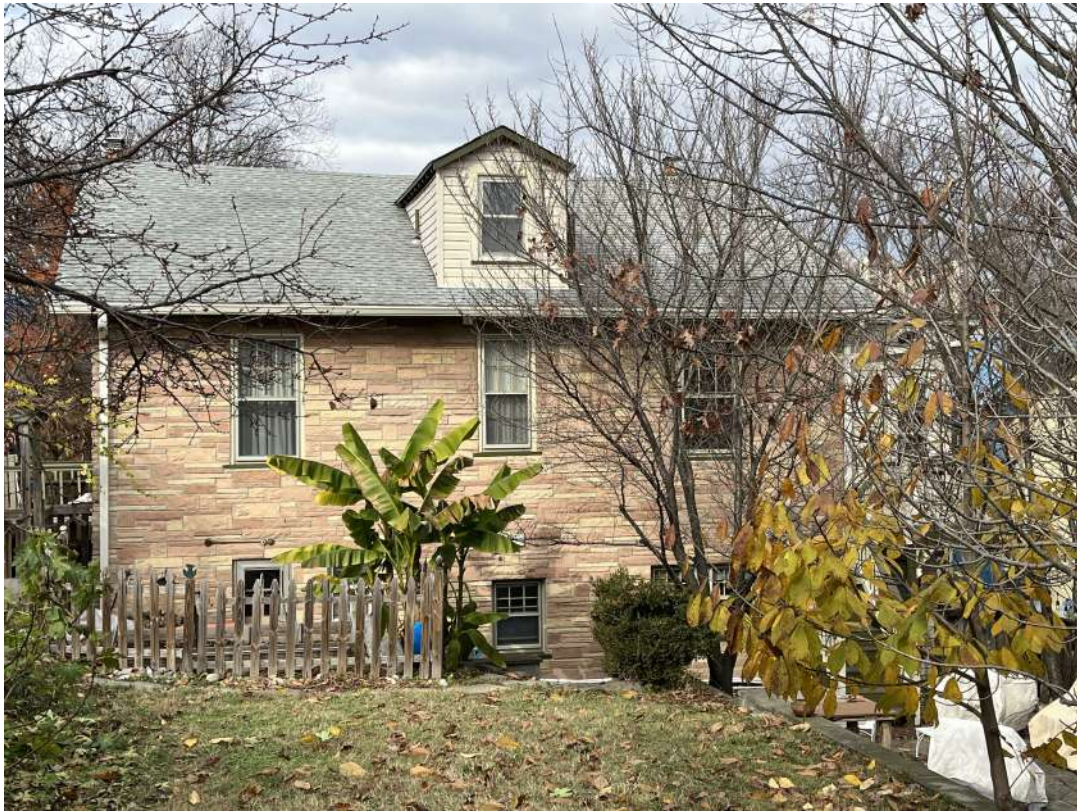
Detail: 51 WALNUT AVE. REAR
