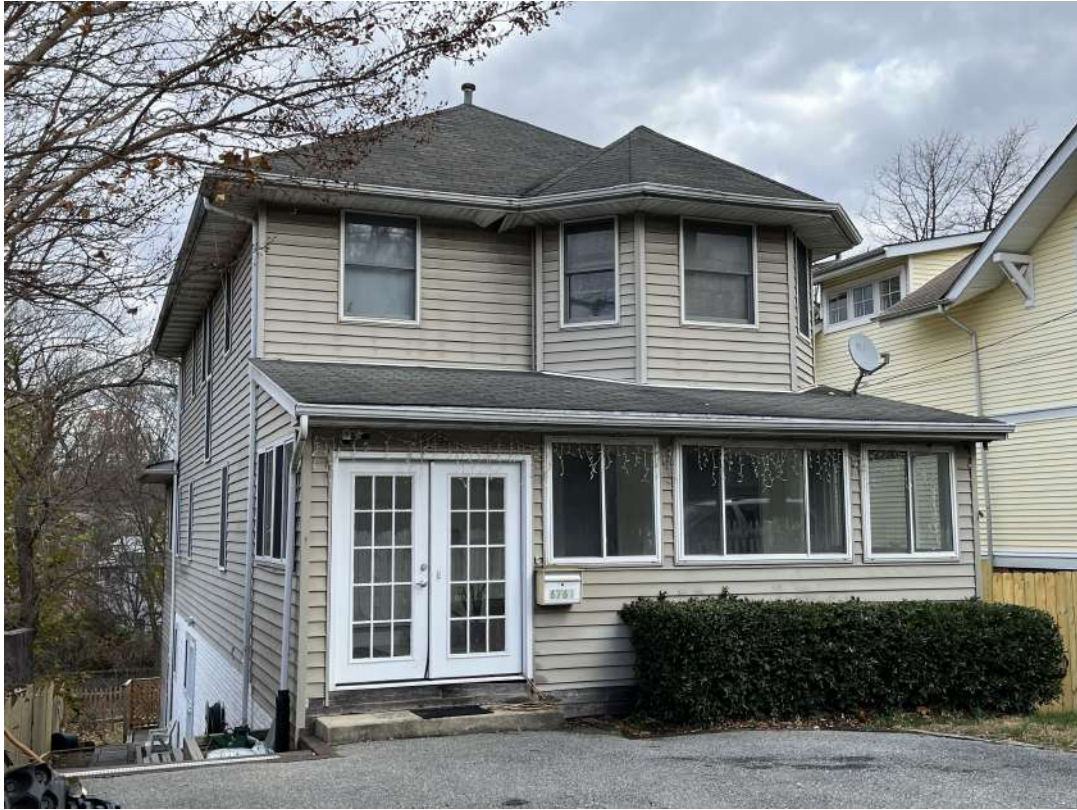
Detail: CONTEXT: 6761 EASTERN AVE.
