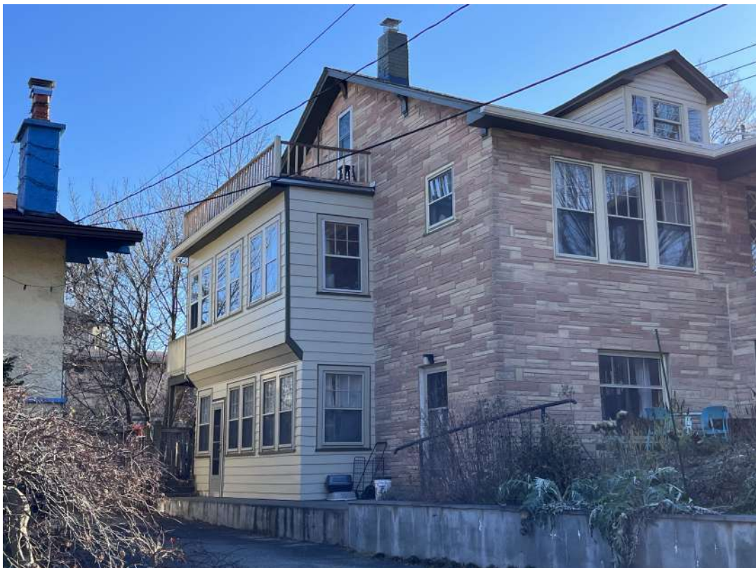
Detail: 51 WALNUT AVE. NORTH-EAST CORNER
