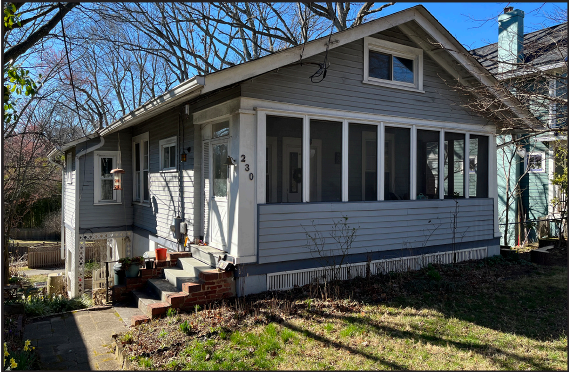
Detail: 230 Park Avenue-Subject-Front / Left (Southeast) side
