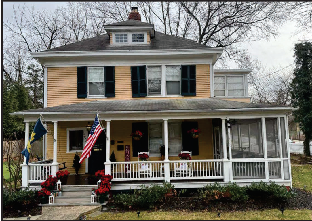
Figure 2. This photo provided by the applicant shows the roof's existing three-tab shingles to be replaced.
