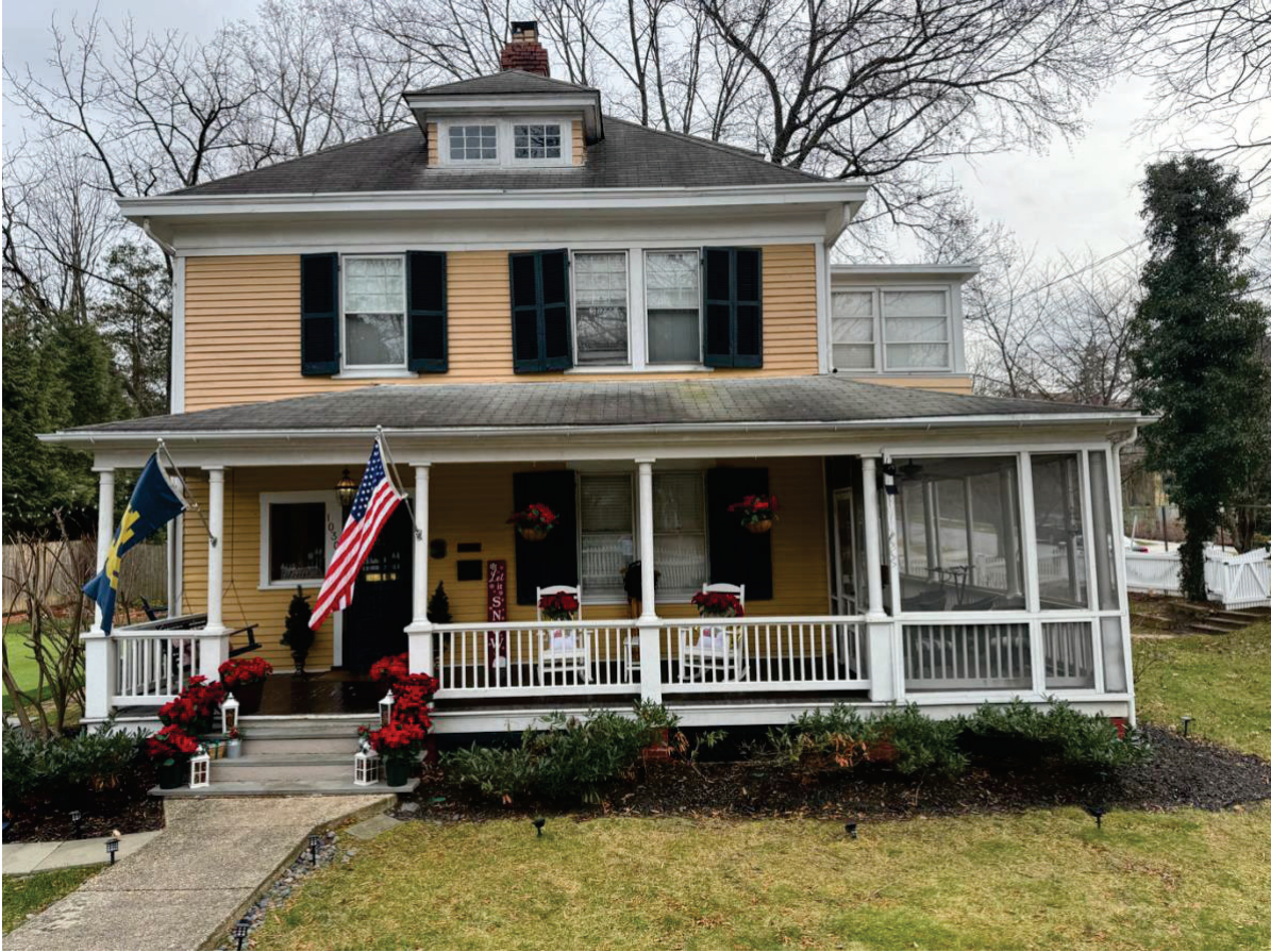
Kensington Mayor's House 10301 Armory Ave Kensington, MD 20895 Work Item #2 – New Roof
