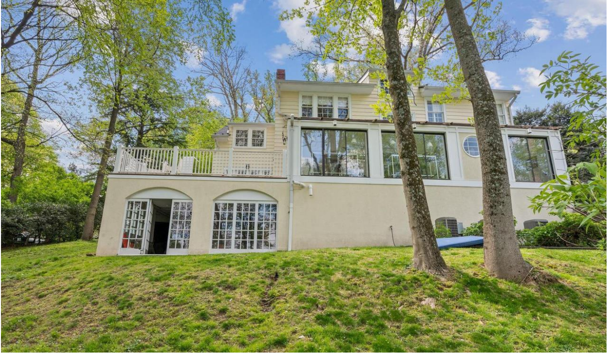
Figure 2: There is currently no deck to the rear of the existing non-historic addition.
