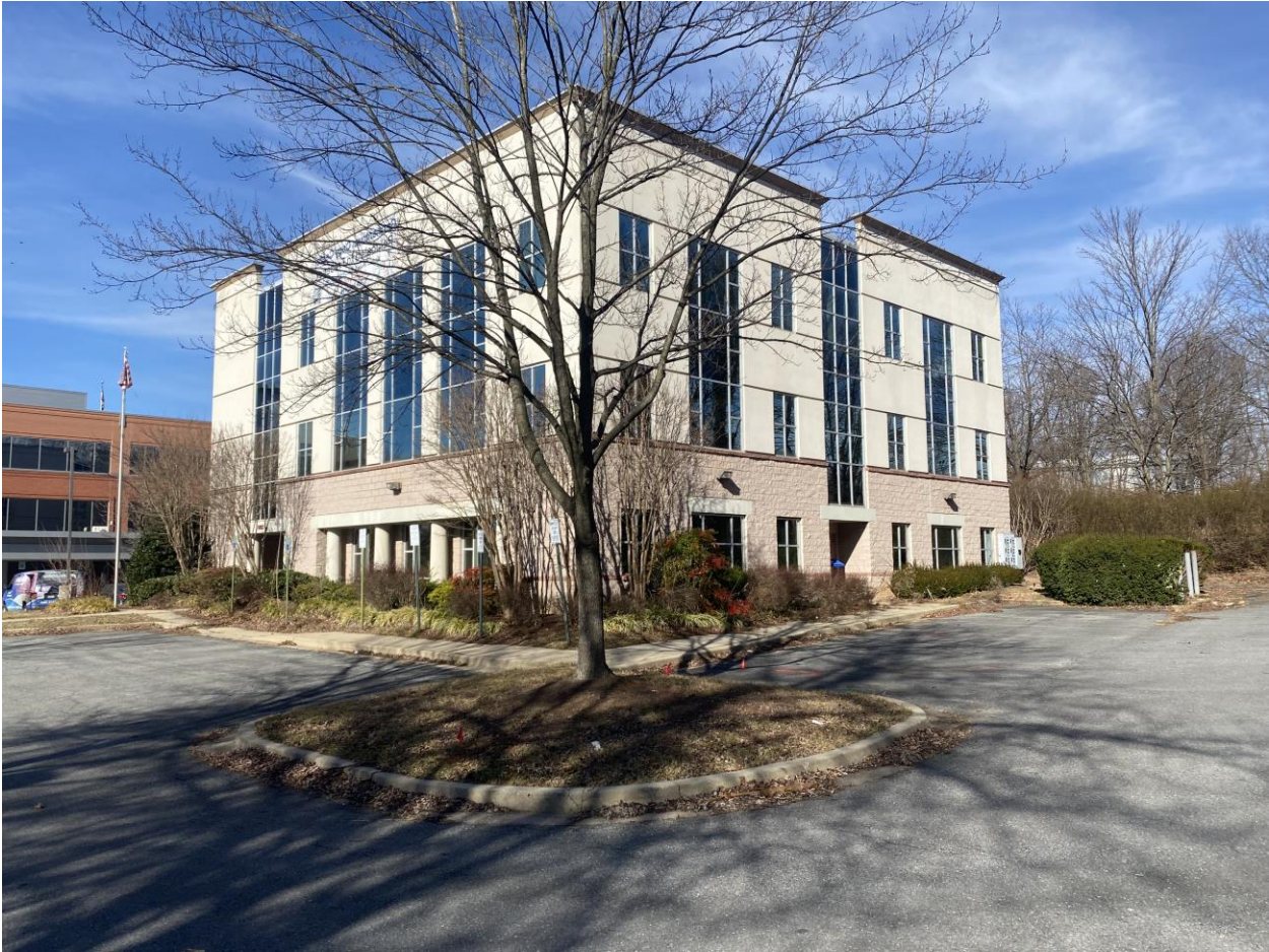
Fig. 4: The subject building proposed for demolition.
