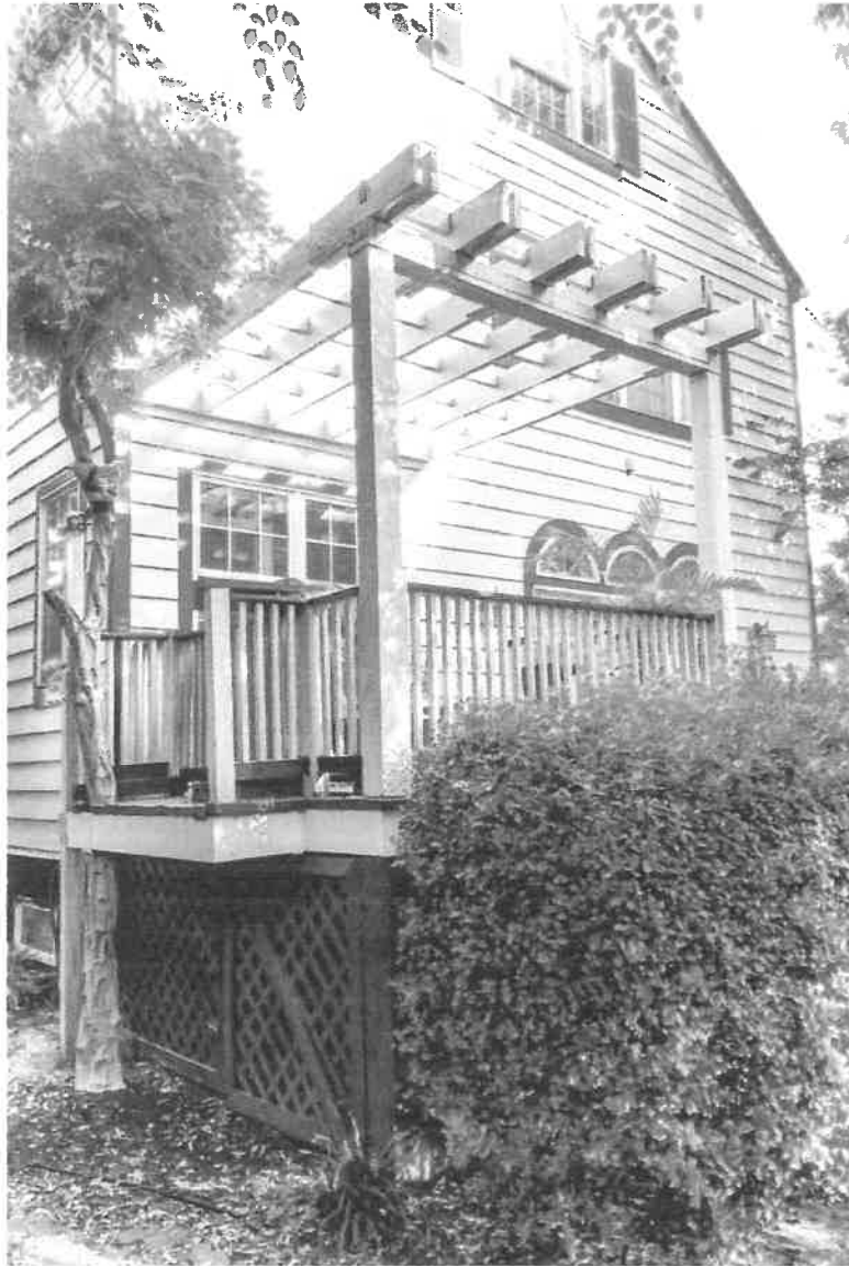
SOUTH ELEVATION OF DECK - DEC. 2023
