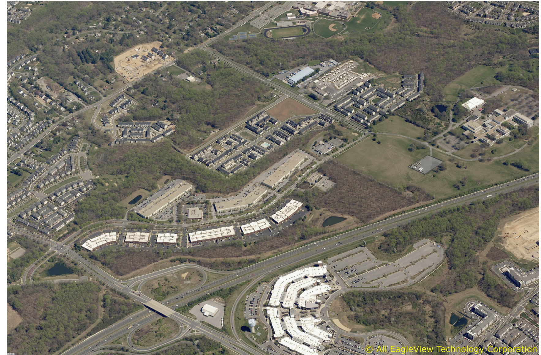
Flex buildings along Gateway Center Drive
