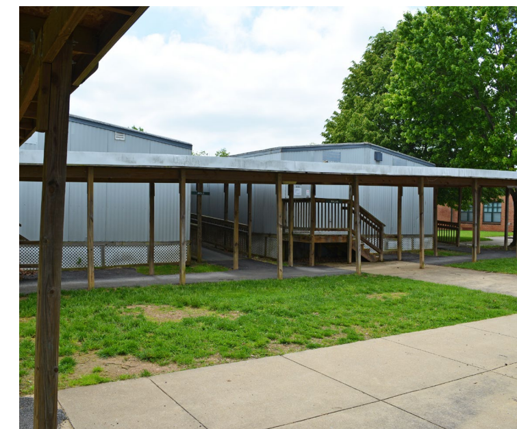
Portables at Clarksburg Elementary School
