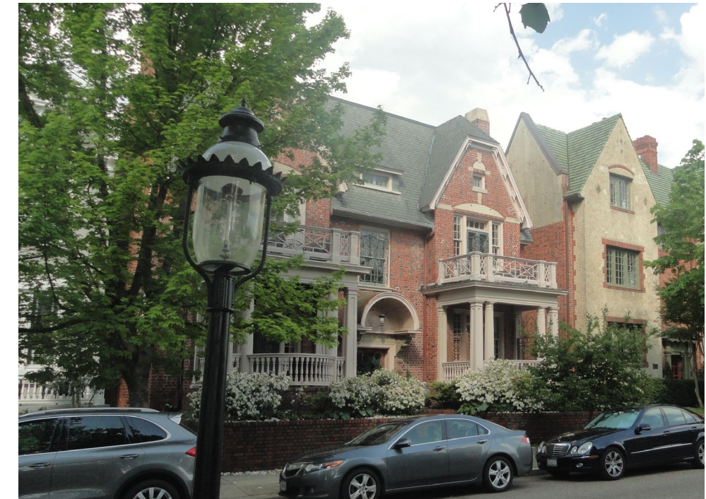
Four-plex apartment building, Richmond
