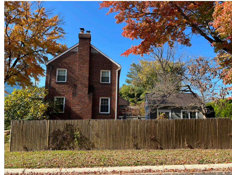
ADU behind single-family home, Bethesda
