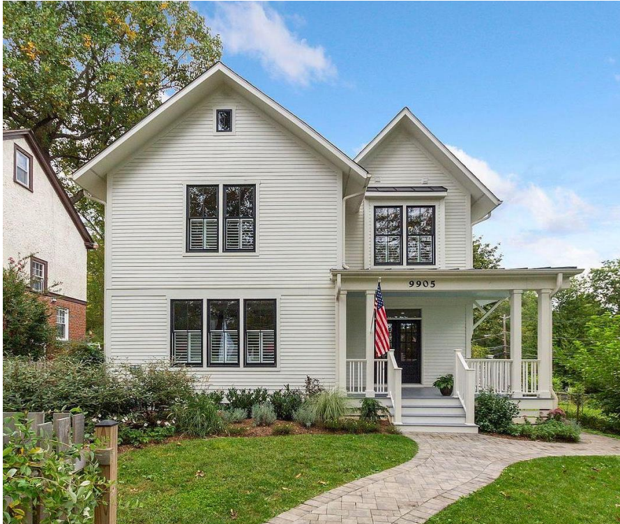
Figure 5: Infill house at 9905 Capitol View Ave. (approved by the HPC in 2015).
