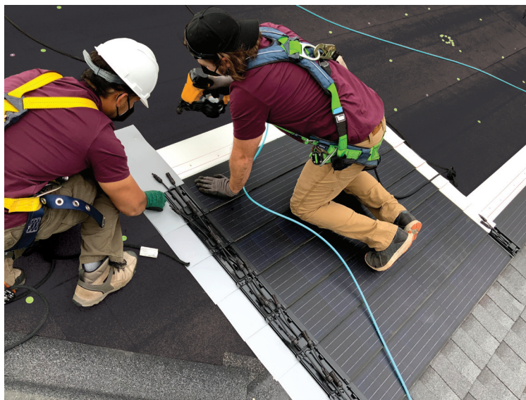
Figure 14. Step Flaps going up the column
