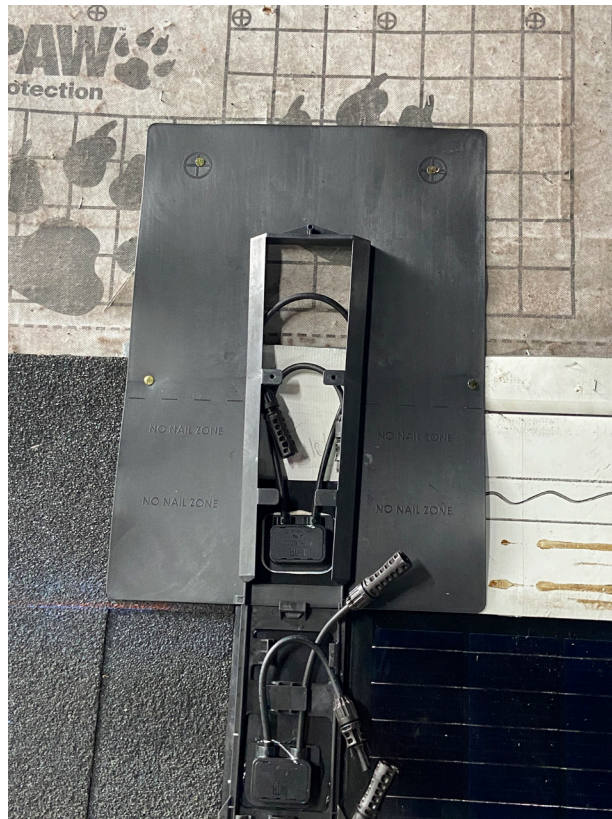
Figure 22. Nail Top Flashing
