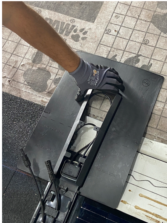
Figure 21. Align Top Flashing
