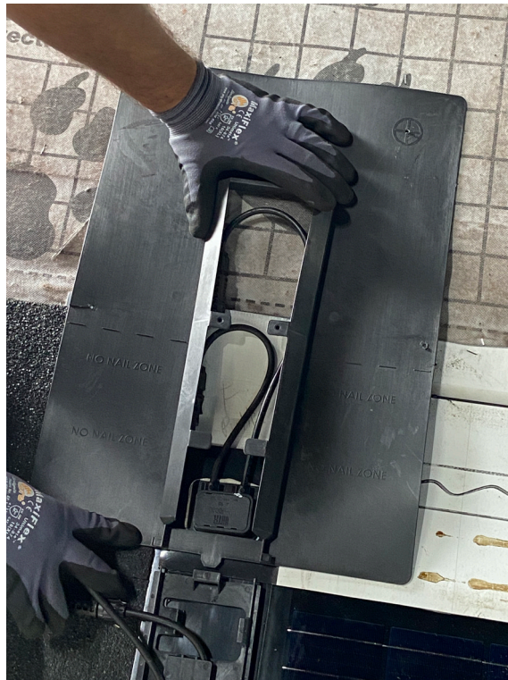
Figure 20. Position Top Flashing
