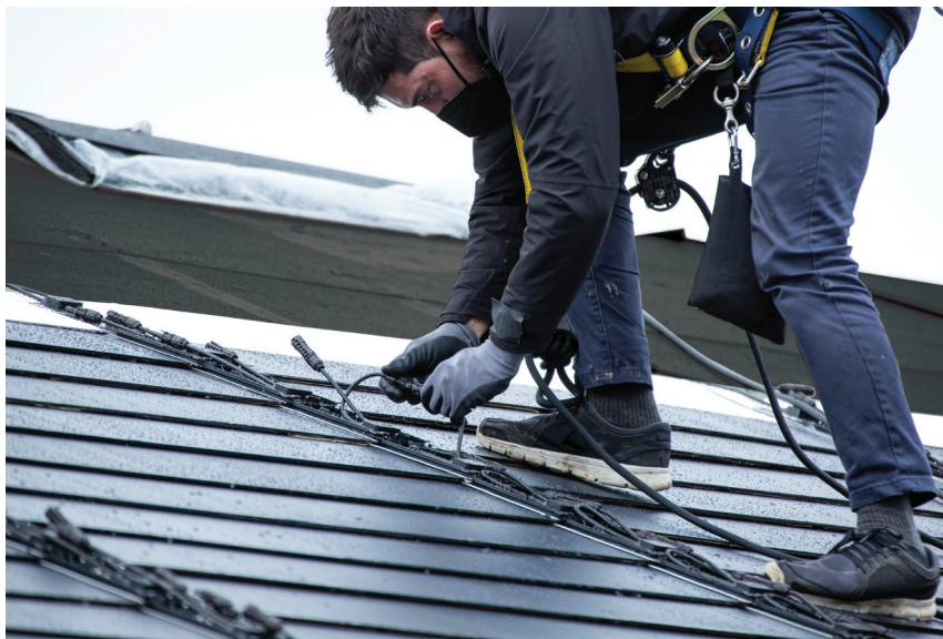
Figure 23. Connect Solar Shingles
