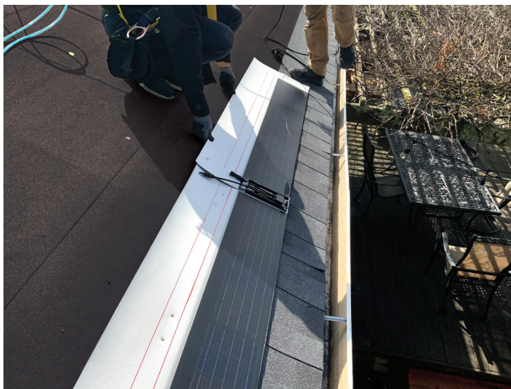
Figure 12. Install next Solar Shingle
