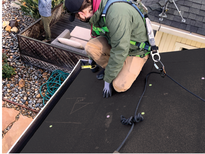
Figure 6. Locate array starting point
