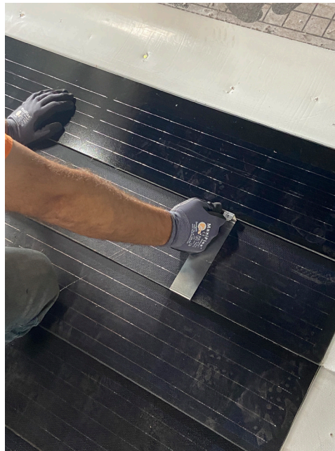
Figure 15. Next Solar Shingle going up the column
