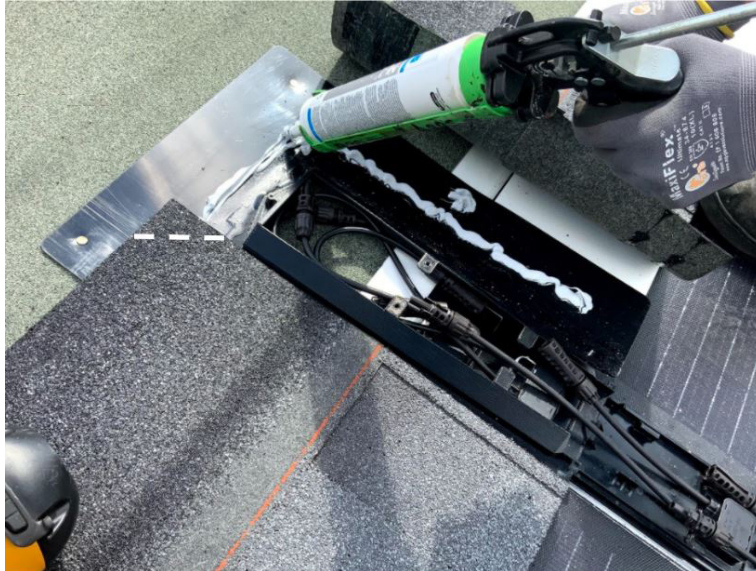
Figure 30. Apply sealant to Top Flashing base
