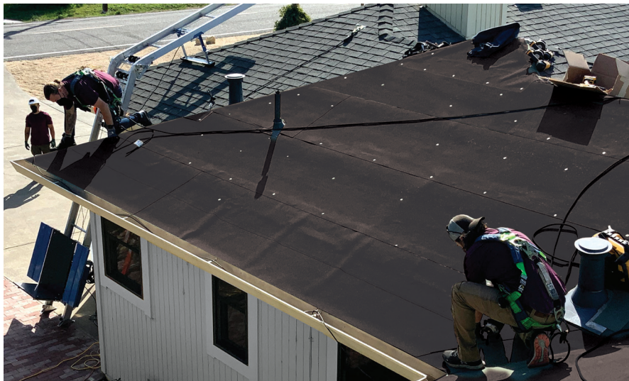
Figure 3. Install roofing underlayment
