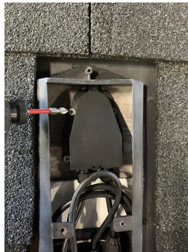
Figure 34. Installing Pass Through Device
