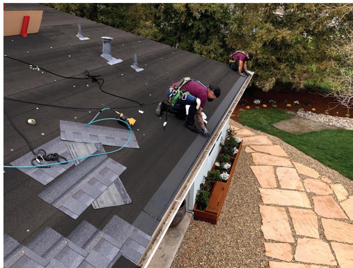
Figure 7. Bottom course of roofing shingles
