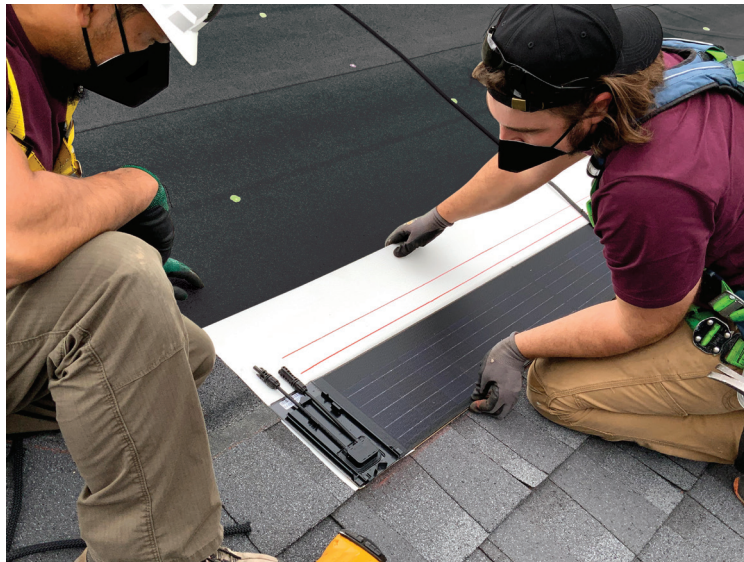
Figure 11. Install first Solar Shingle
