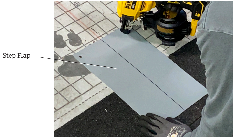
Figure 10. Nail Step Flap in place
