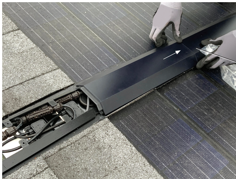
Figure 25. Use built-in wire clip features to secure wires
