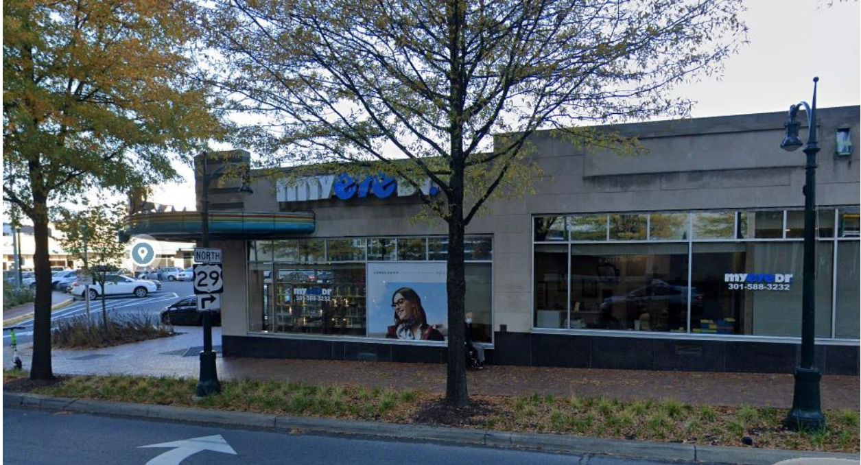
Figure 3: The existing sign facing Georgia Ave. (to be removed) is identical to the one proposed in this HAWP.
