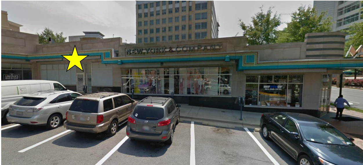
Figure 2: The applicant proposes to install signage above the storefront behind the yellow star.
