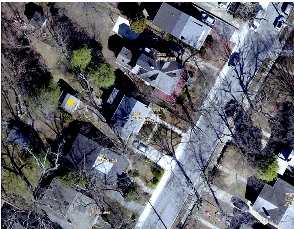
Figure 2: A closer aerial view of the garage at the subject property.
