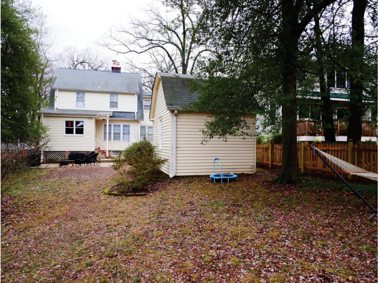
Right and rear elevations and holly tree to be removed in rear.
