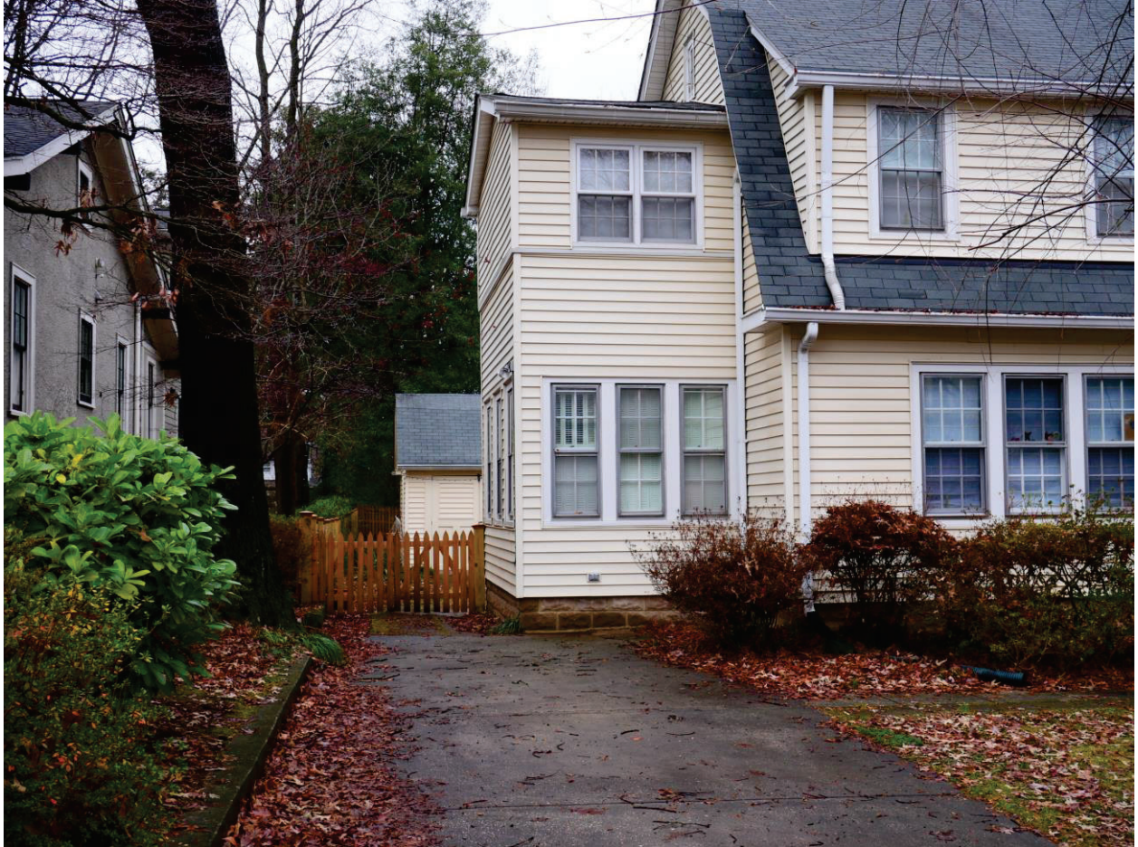
Accessory structure from right of way.
