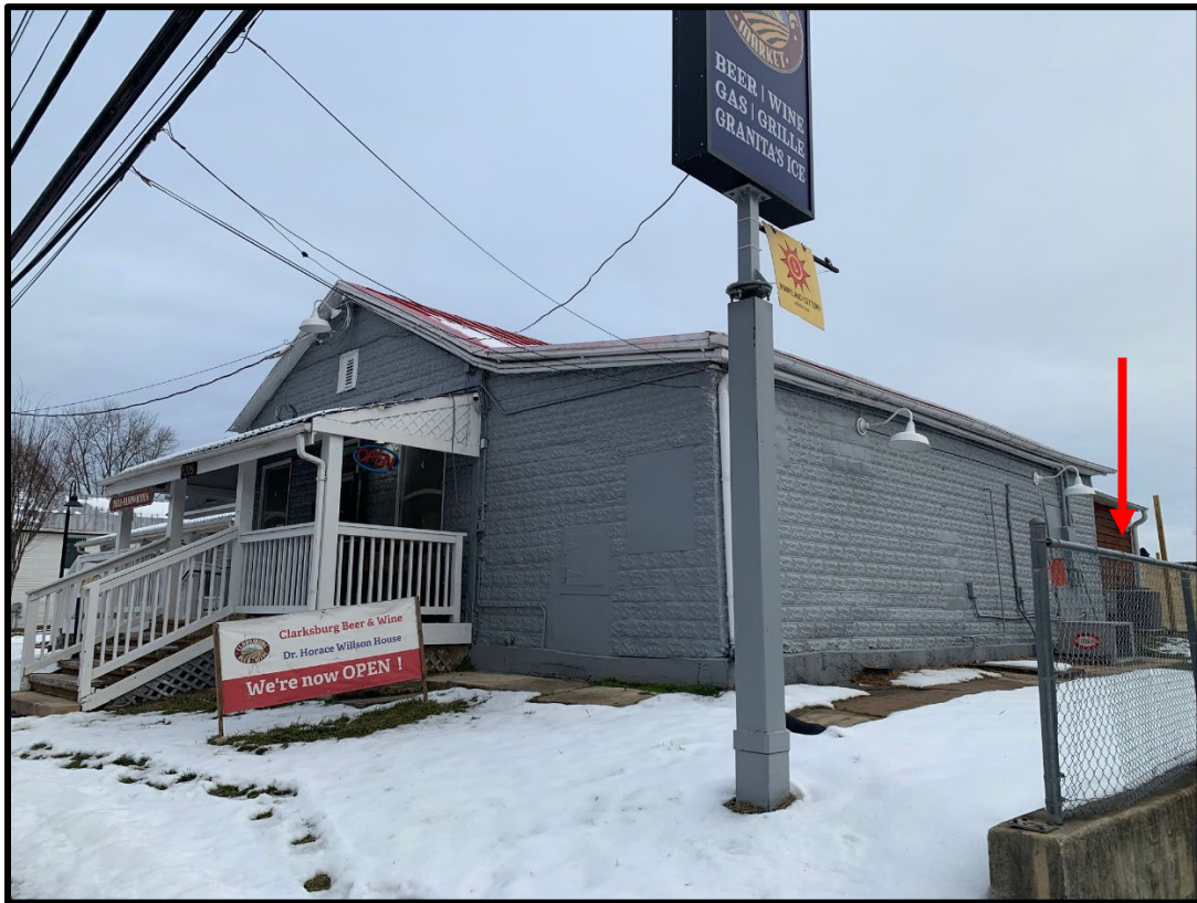
Figure 2: The front and right-side elevations of the Clarksburg Market as viewed from the right of way. The proposed door location is indicated with a red arrow.
