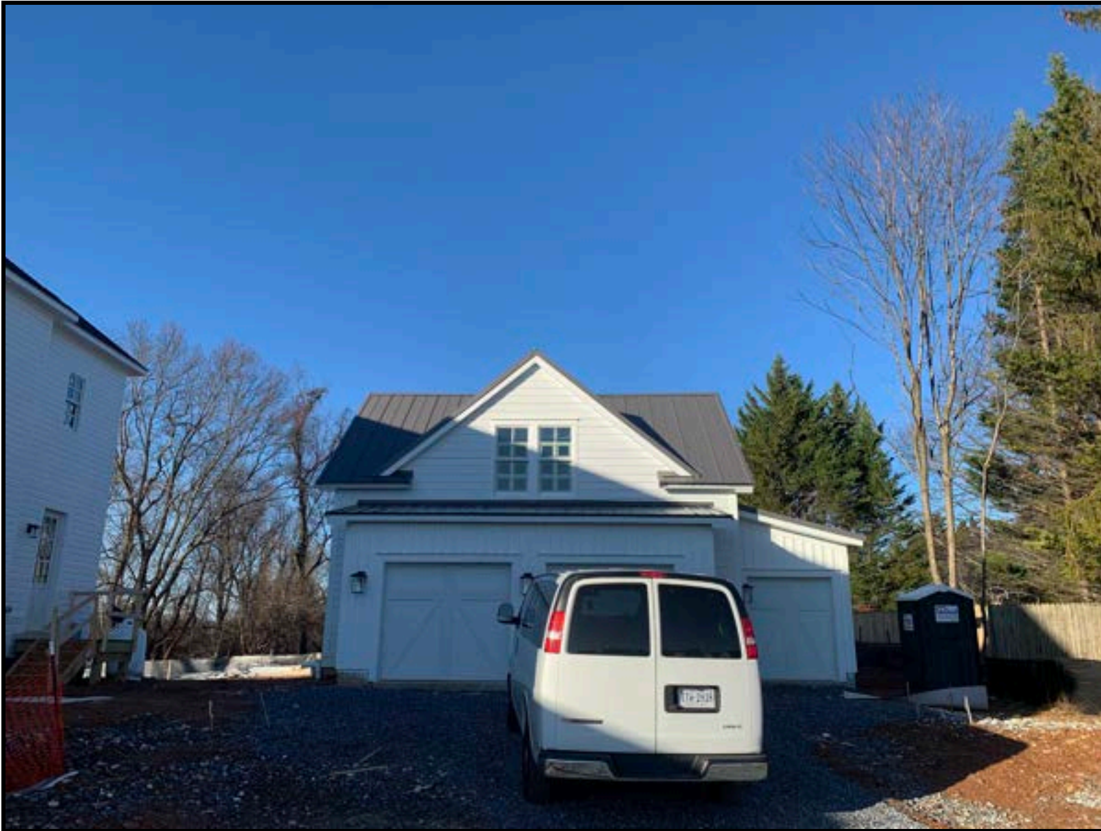
Figure 18: The front elevation of the garage on January 11, 2024.
