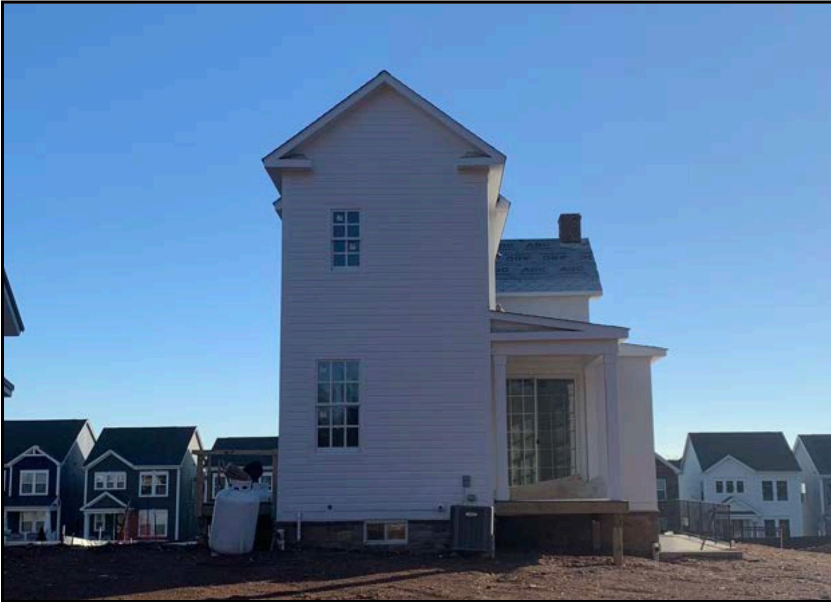
Figure 15: The rear elevation on January 11, 2024.
