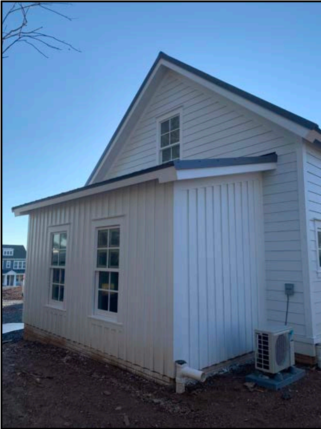
Figure 21: The right side of the garage on January 11, 2024.
