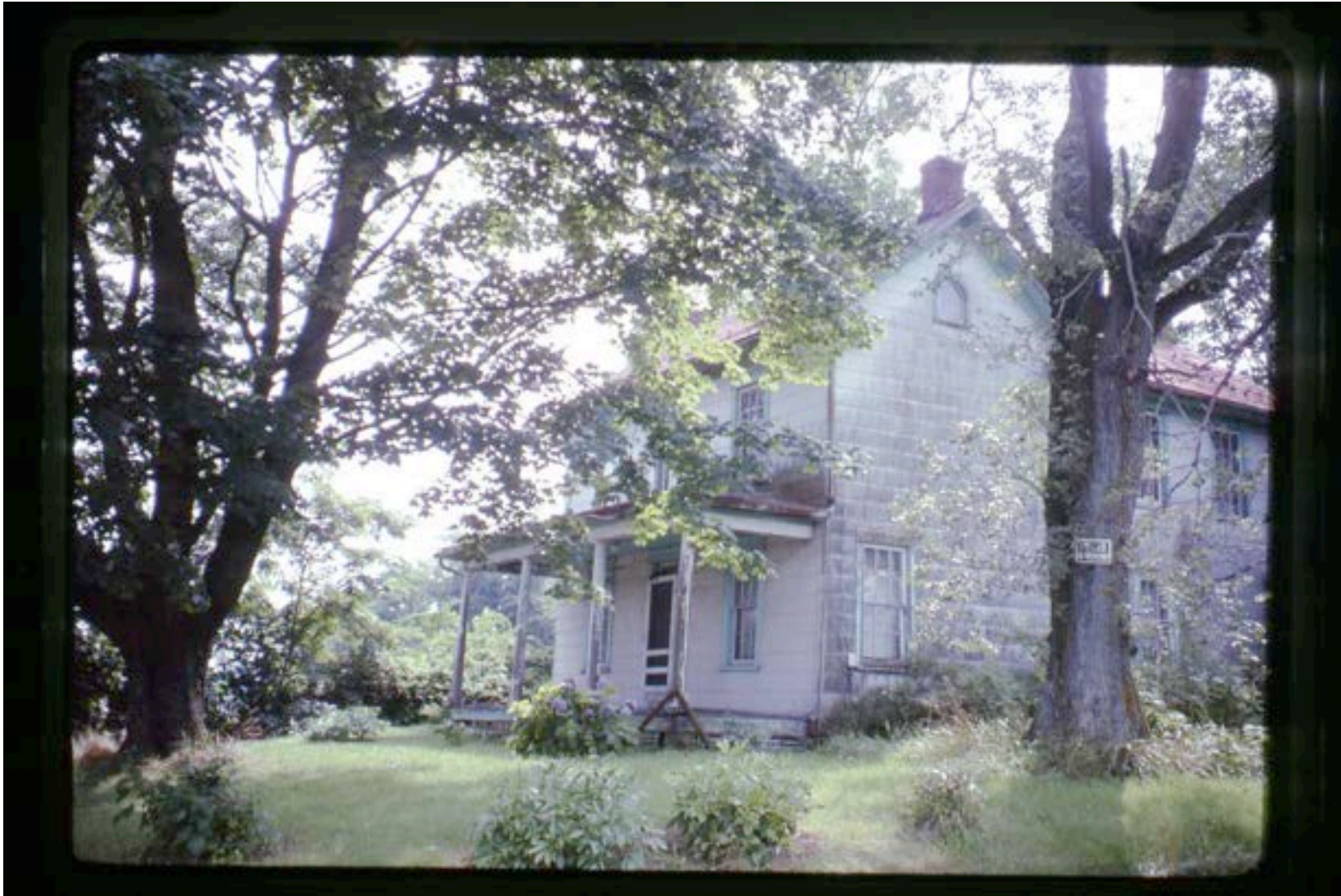
Figure 12: The site will be regraded near the front porch to approximate the grading shown in this archival photo of the Cephas Summers House.
