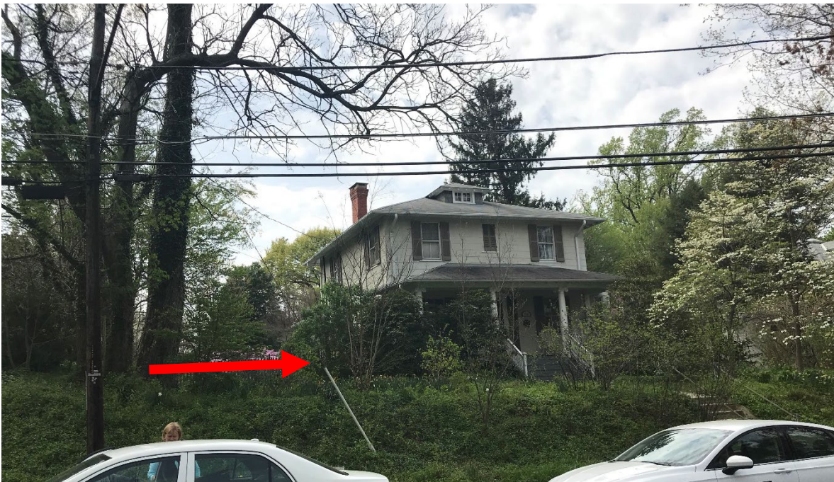
Figure 2: This 2019 photo shows the front elevation of 10922 Montrose Ave. The proposed generator location is indicated with an arrow and will be minimally visible from the right of way.
