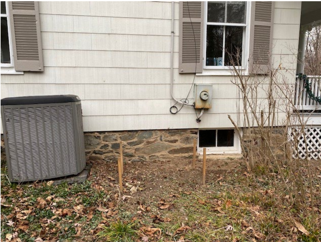
Figure 4: The proposed generator location is indicated with stakes in this photo.
