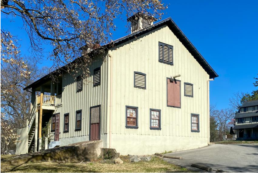
Figure 2: east elevation of the carriage house, showing the access to the hay loft.
