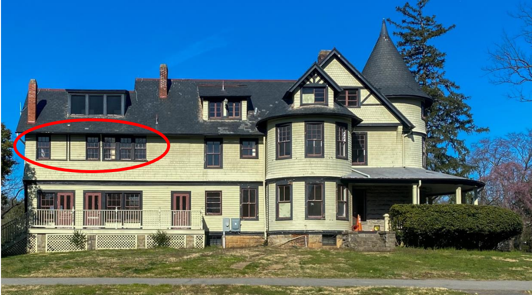
Figure 13: Existing east elevation. Altered windows circled in red.
