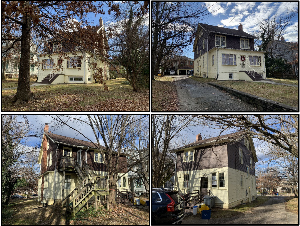
Figure 2: From top left and continuing clockwise: the front and right-side elevations; the front and left-side elevations; the rear and left-side elevations; and the rear and right-side elevations.
