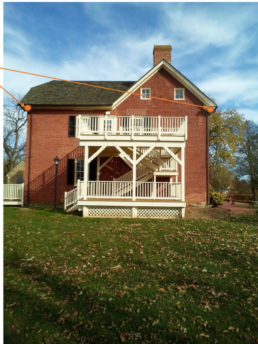
Figure 4: The applicant provided this diagram to show the locations of the cameras at the left side elevation of the Manor House.
