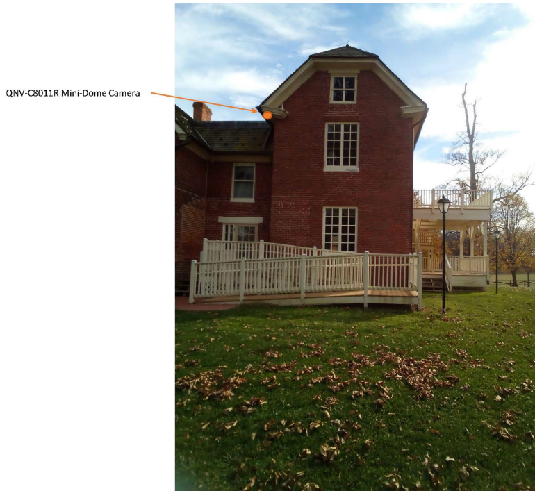
Figure 5: The applicant provided this diagram to show the locations of the camera on the rear elevation of the Manor House.
