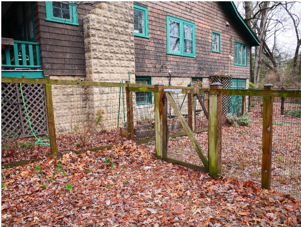
Figure 4. The wood and wire fence in the side yard.
