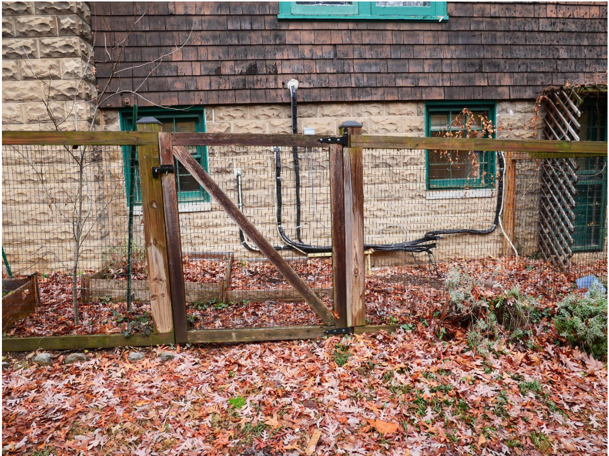
Wood and wire fence in side yard.
