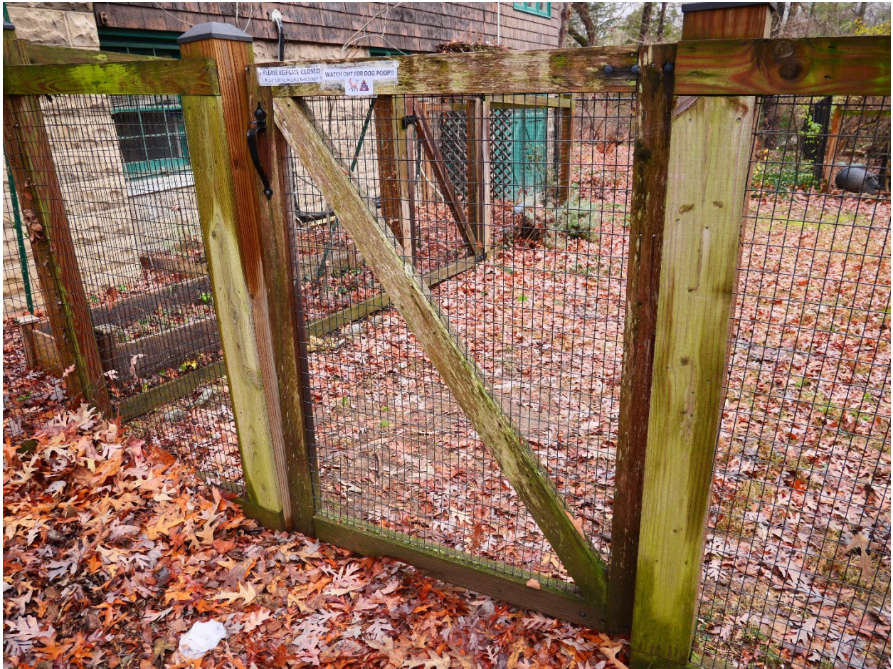
Wood and wire fence in side yard.
