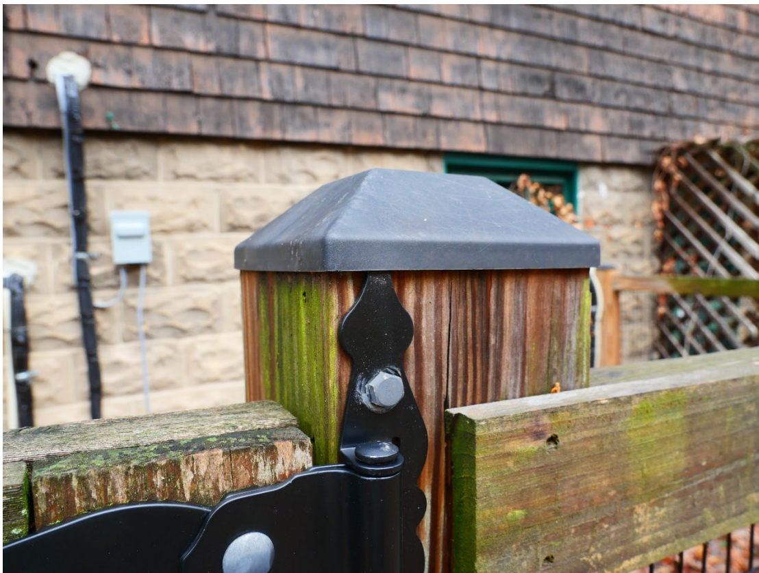
Figure 6. A detail of the caps on the posts of the wood and wire fence.
