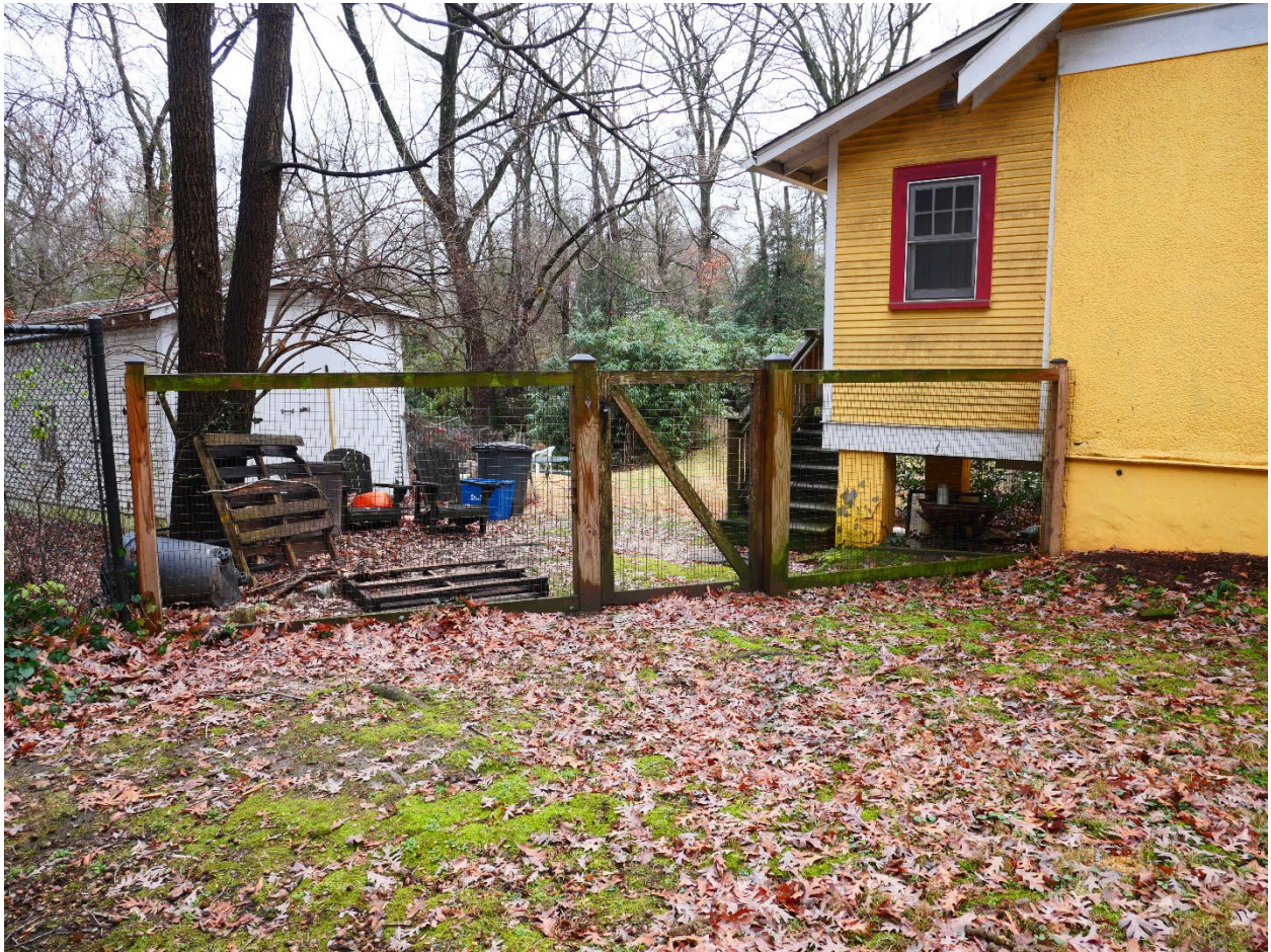
Wood and wire fence that connects to 7401 Baltimore Ave.
