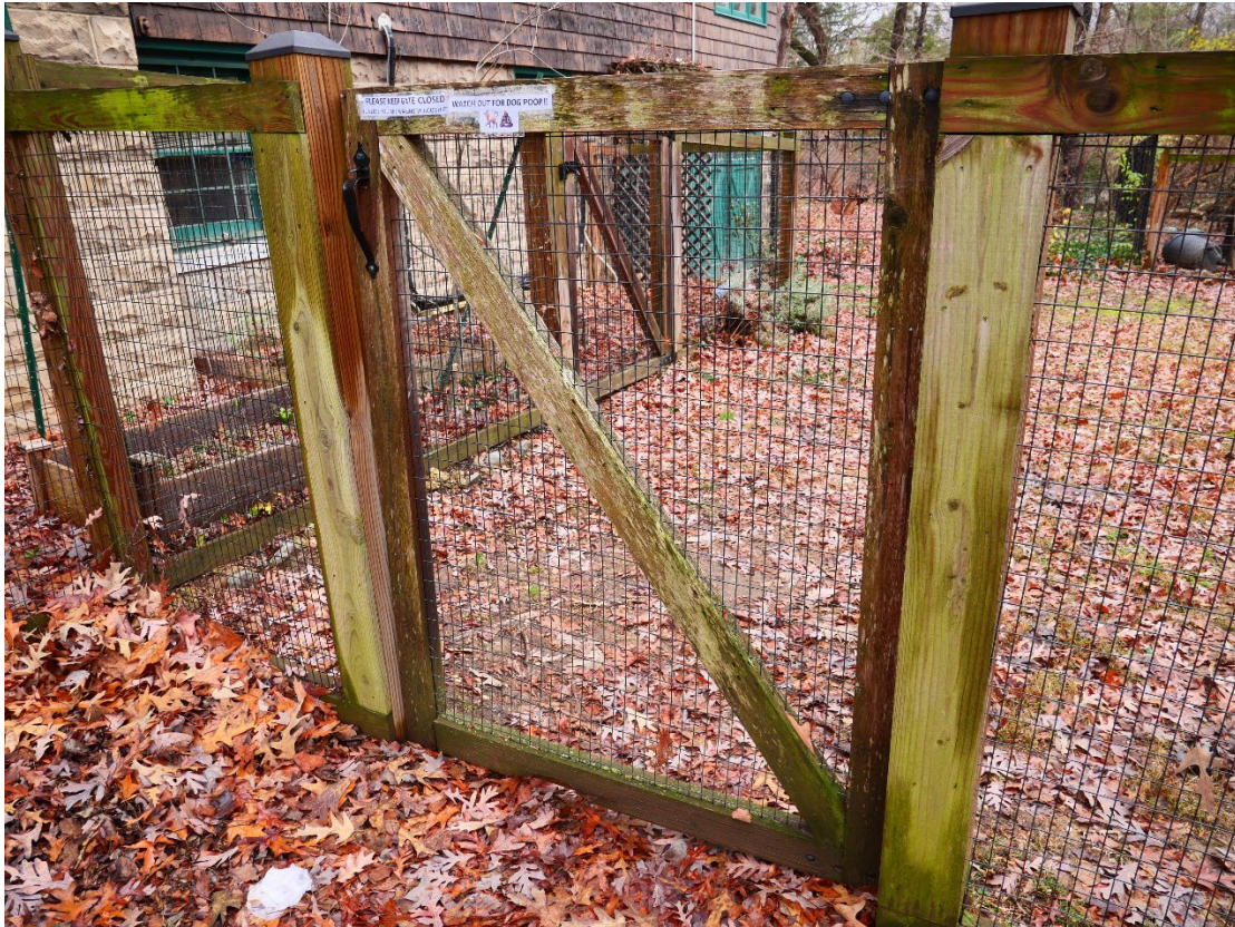
Figure 5. A detail of the wood and wire fence.
