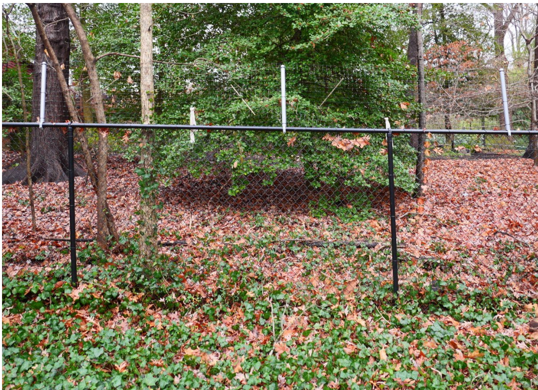
Figure 8. The chain link fence on the north property line with two-foot tall metal and mesh extenders to create an approximately eight foot tall fence.
