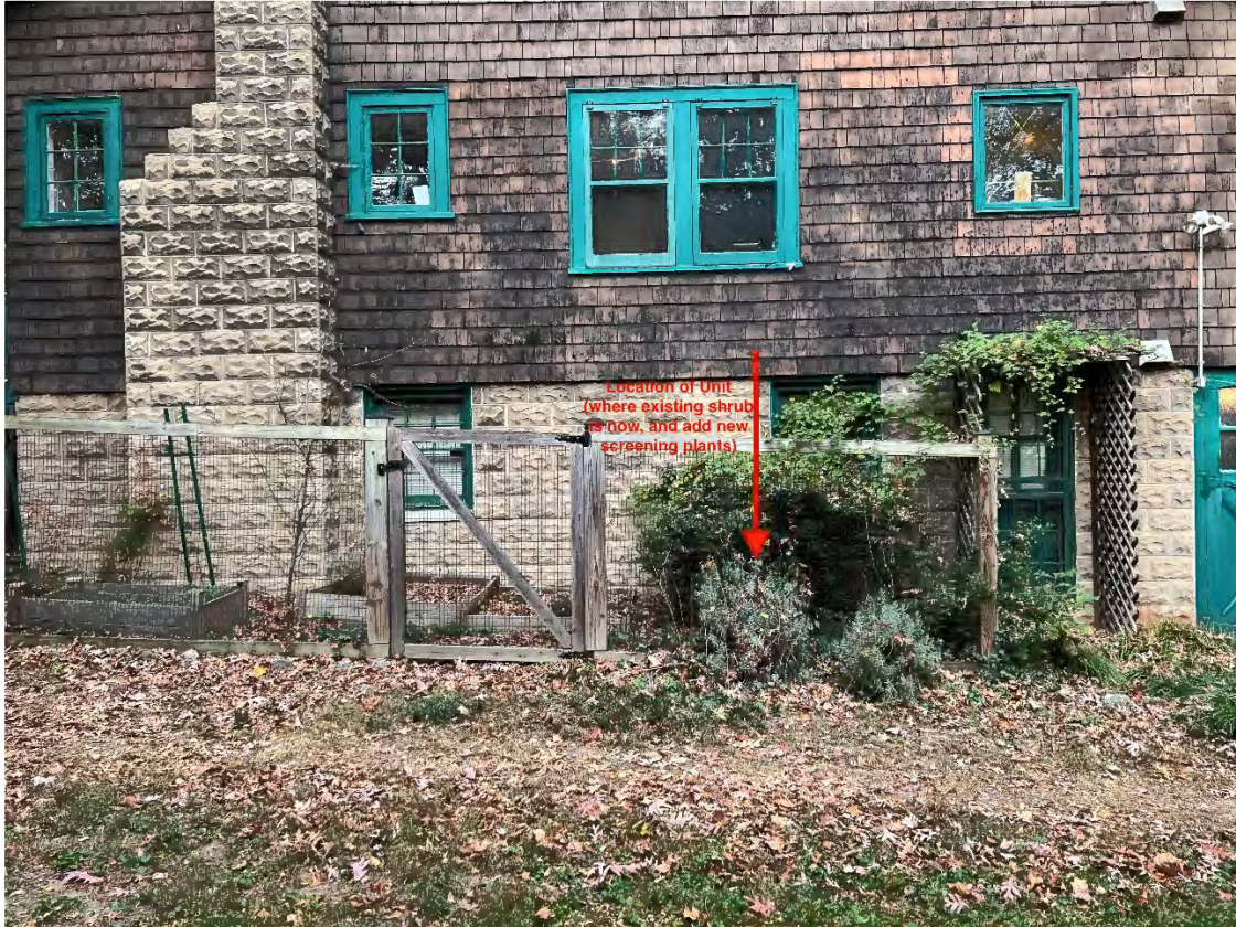
Figure 3: The applicant provided this photo to show the location the condenser.
