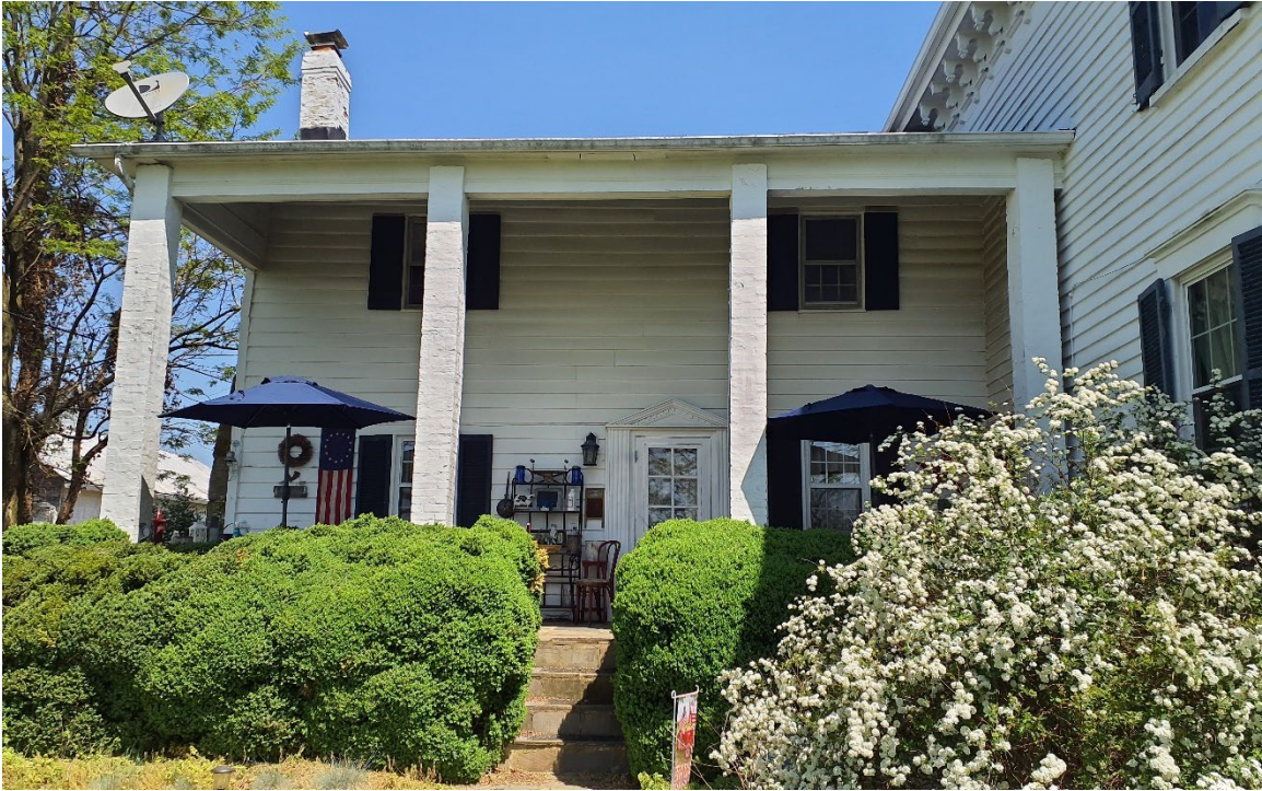
Figure 28: Original c.1820 front facade, facing north.
