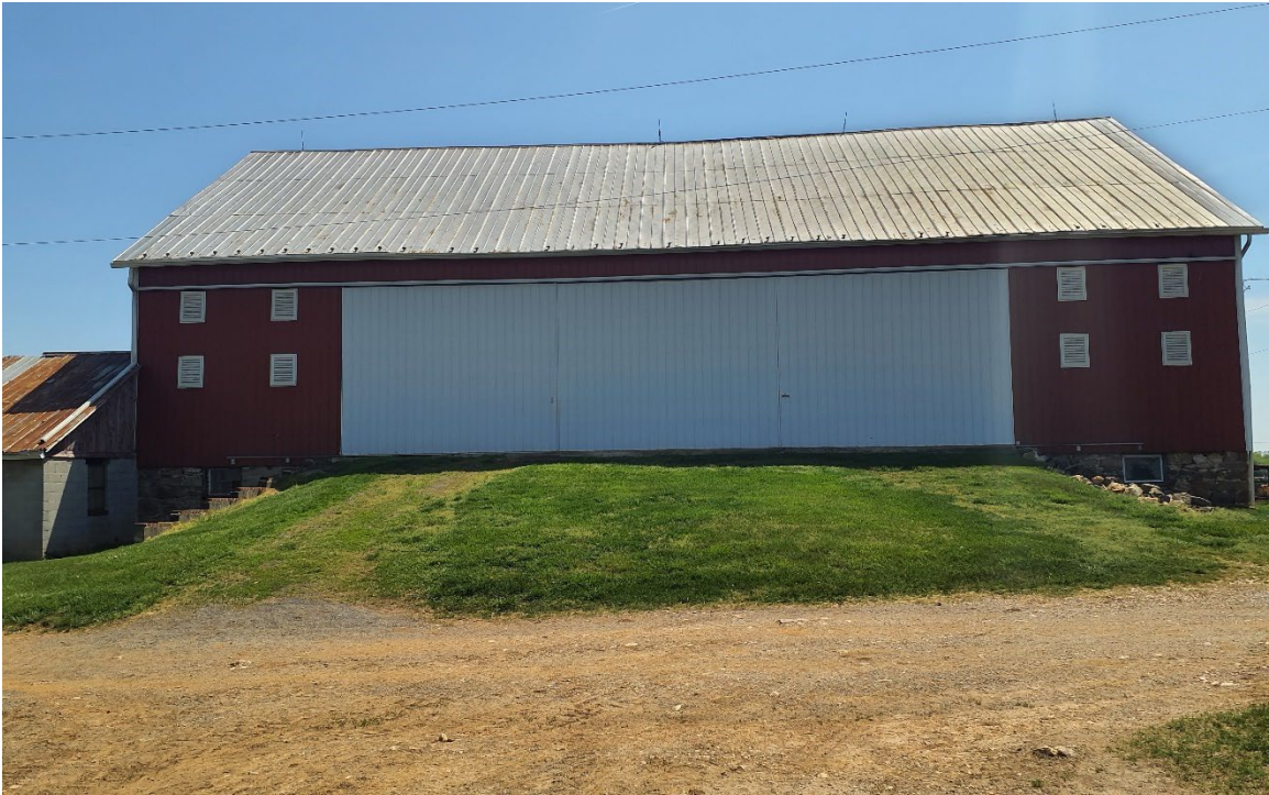
Figure 25: General view of nineteenth century bank barn, facing east.
