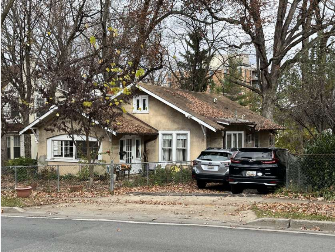
Detail: 46 PHILADELPHIA AVE. SOUTHERN APPROACH
