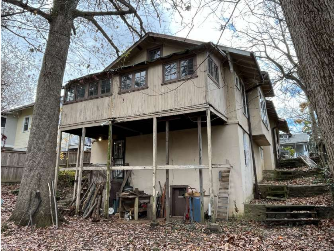
Detail: 46 PHILADELPHIA AVE. REAR-NORTHERN CORNER
