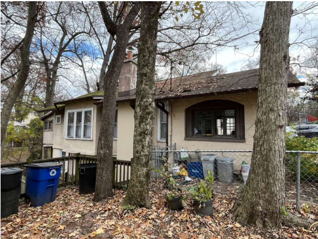
Detail: 46 PHILADELPHIA AVE. NORTH-WEST SIDE
