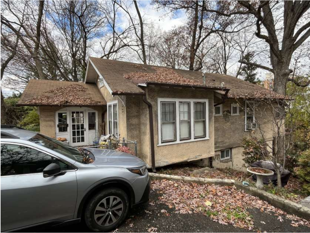
Detail: 46 PHILADELPHIA AVE. SOUTH-EAST SIDE
