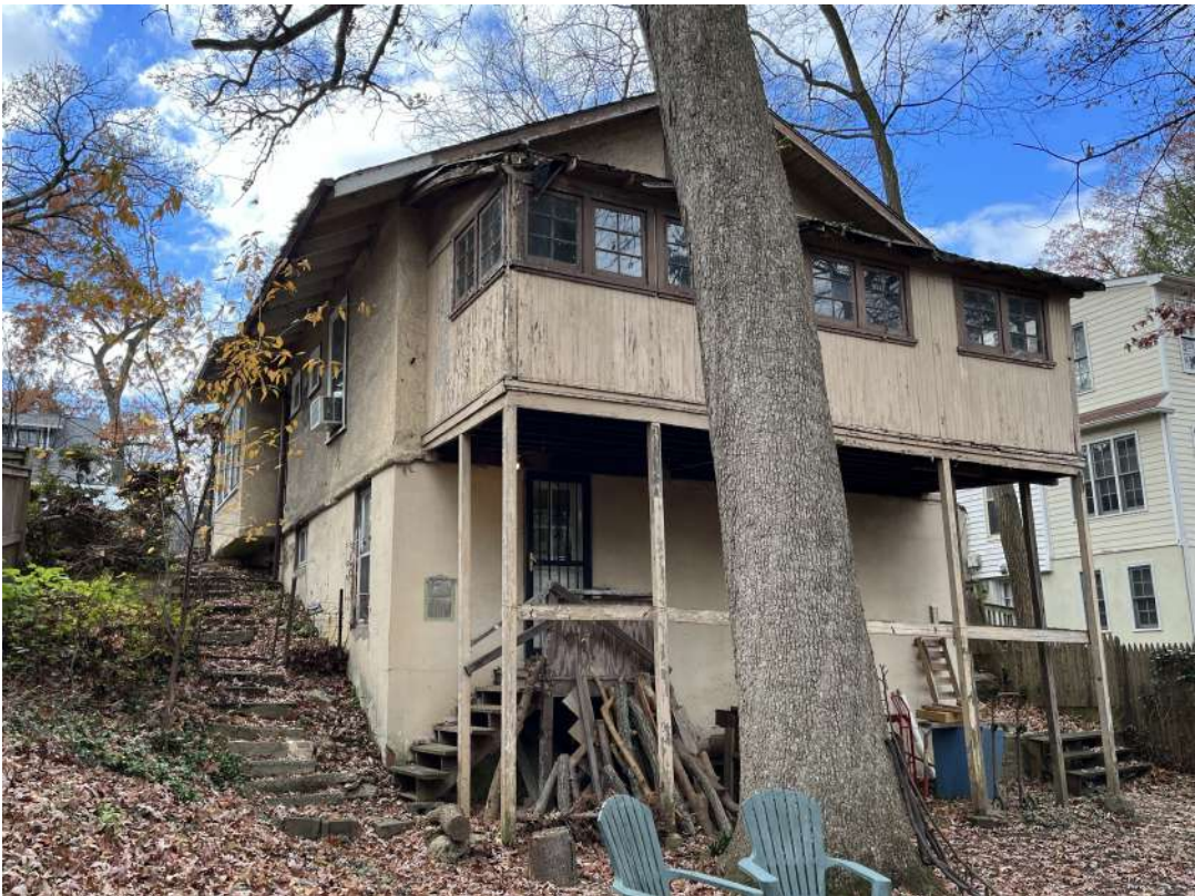
Detail: 46 PHILADELPHIA AVE. REAR-EASTERN CORNER
