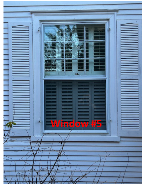
Side View (Facing East from Driveway)
