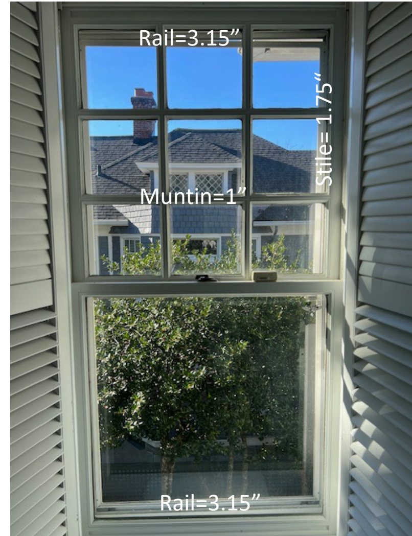
Window #6 – 2 nd Floor Bathroom
