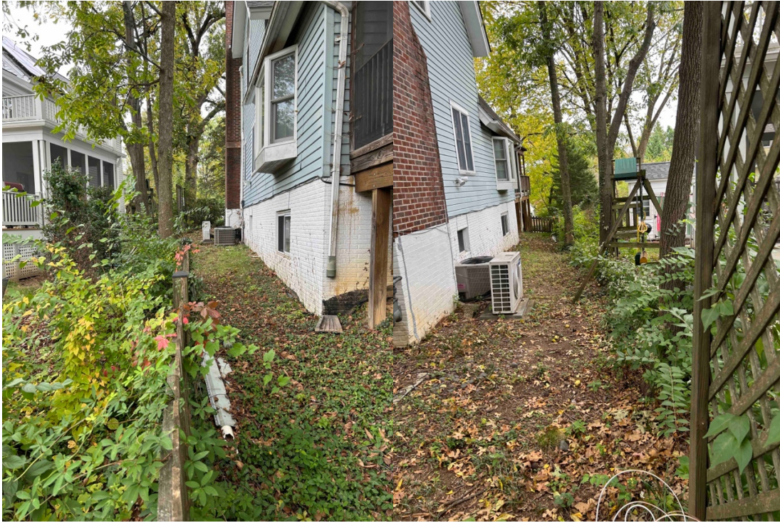
South to North View
