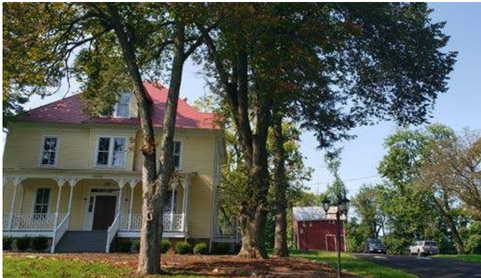
Hammer Hill with Building Site in Background
