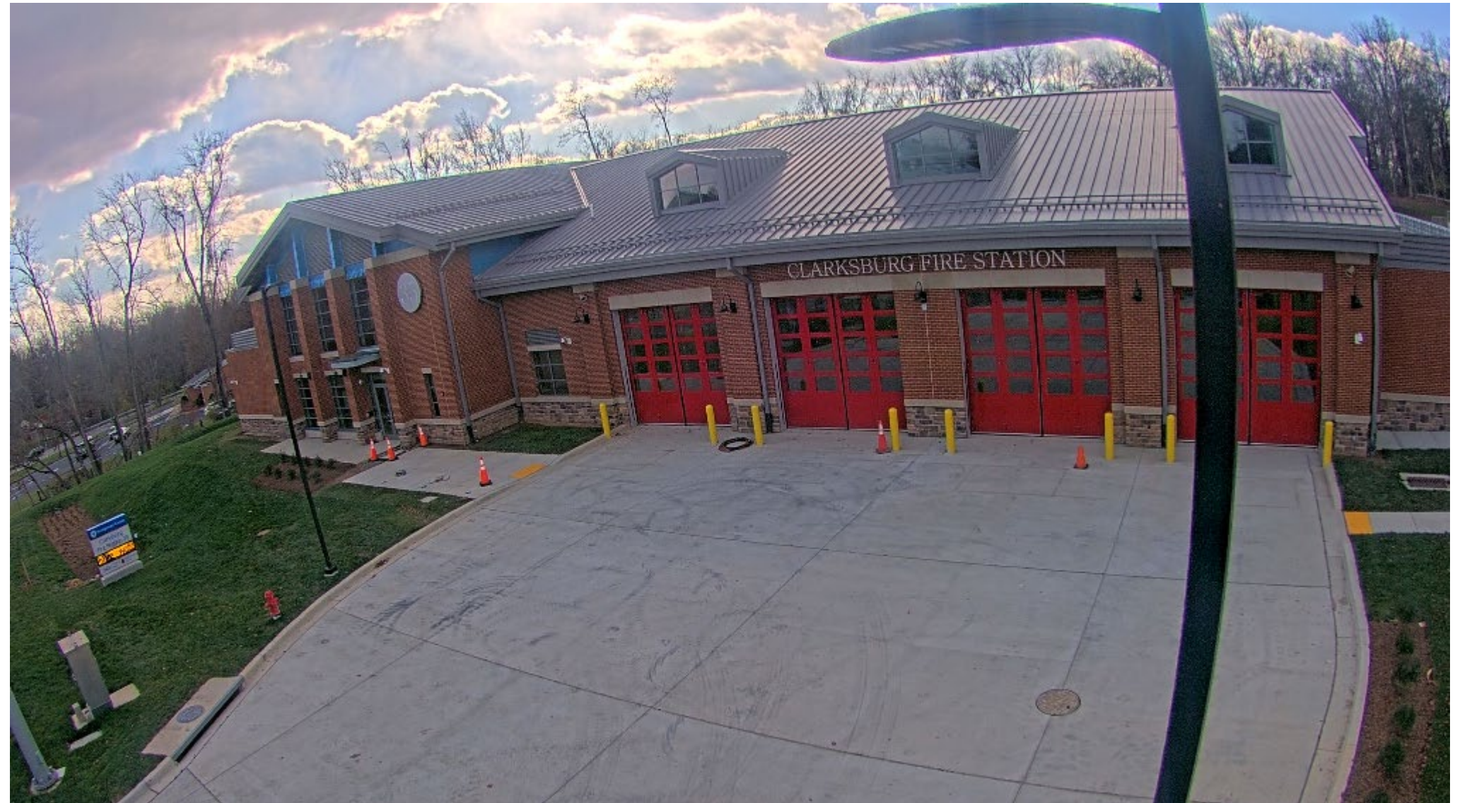
Construction progress as of November 28, 2023. Image source: Montgomery County Department of General Services
