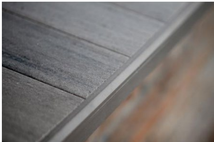
Figure 3: Detail of the chamfer nosing trim.
