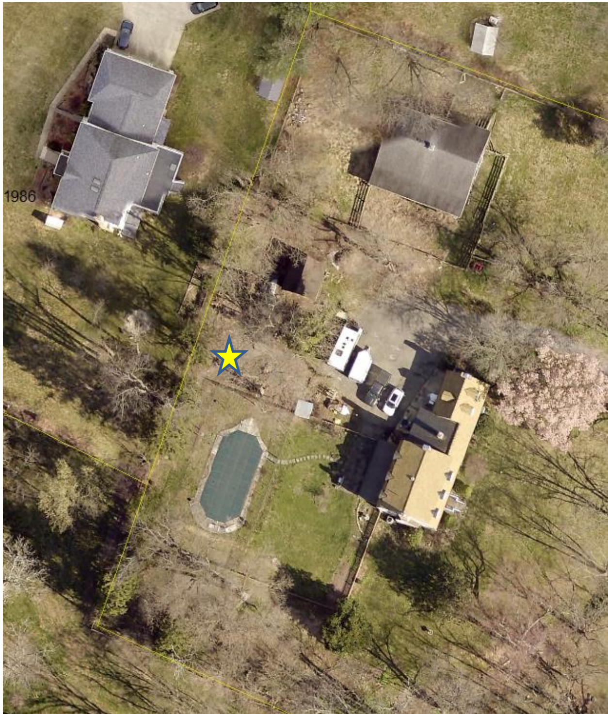
Figure 2: Detail showing the house, pool, barn, log cabin, and proposed shed location.
