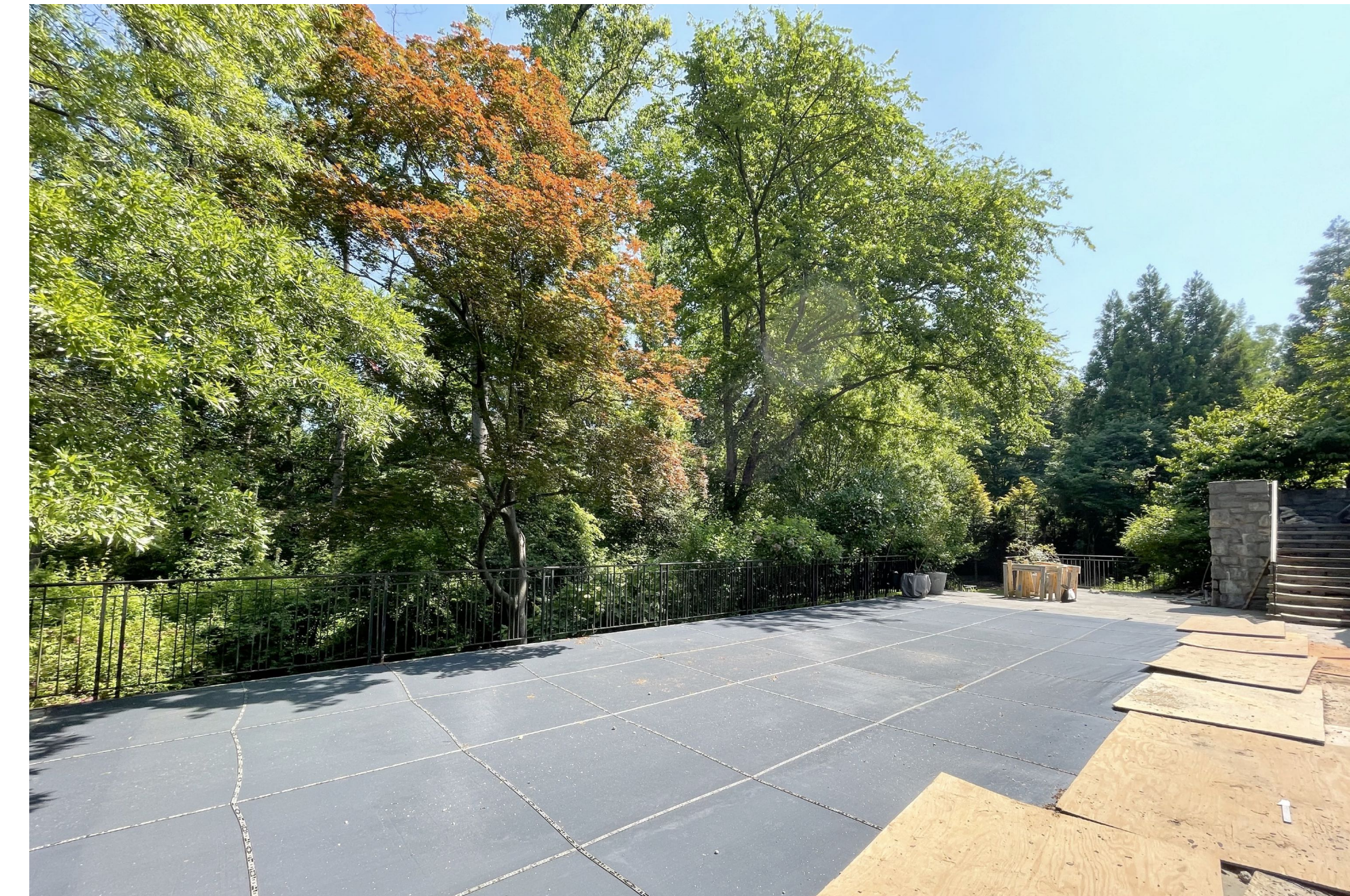
EXISTING POOL TERRACE AND STAIRS TO UPPER TERRACE
