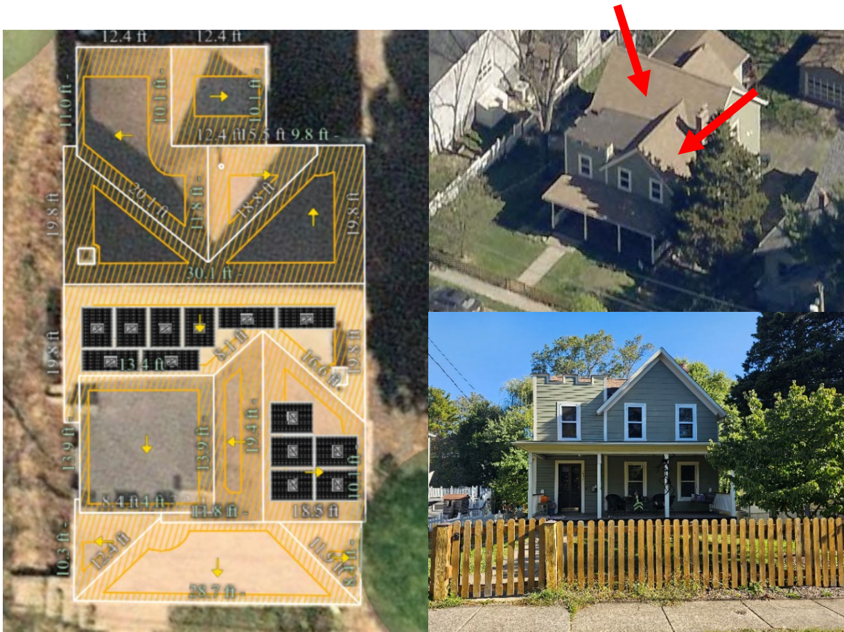
Figure 4: Aerial view showing the location of the solar arrays (left), oblique view with the red arrows pointing to the location of the two arrays (top right), and view of the façade from Takoma Avenue (bottom right). Source: Applicant, ConnectExplorer, and Montgomery Planning.
