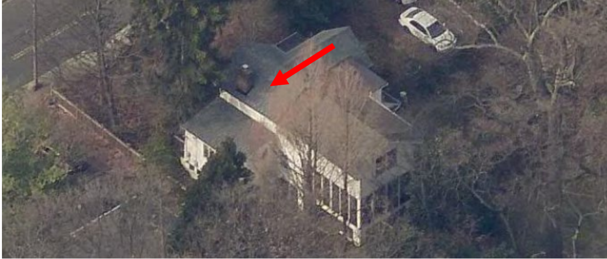
Figure 4: Aerial view showing the rear and side elevations of the subject house. The red arrows point to the locations of the single proposed array on the historic house.
