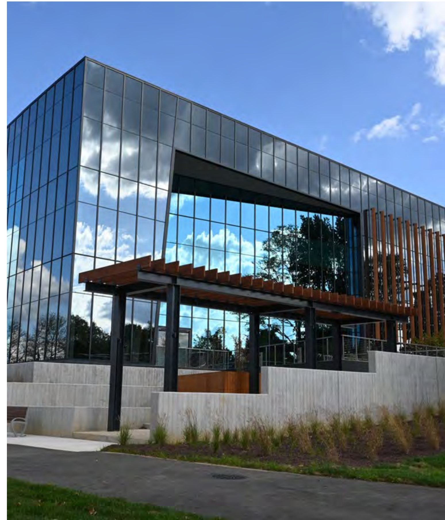
Figure 3: Recently Constructed Building in Life Sciences Center
