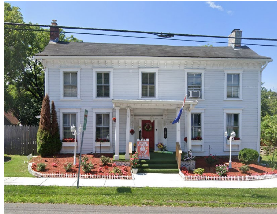
Clark-Waters House, 23346 Frederick Road, 2022. Source: Google Street View
