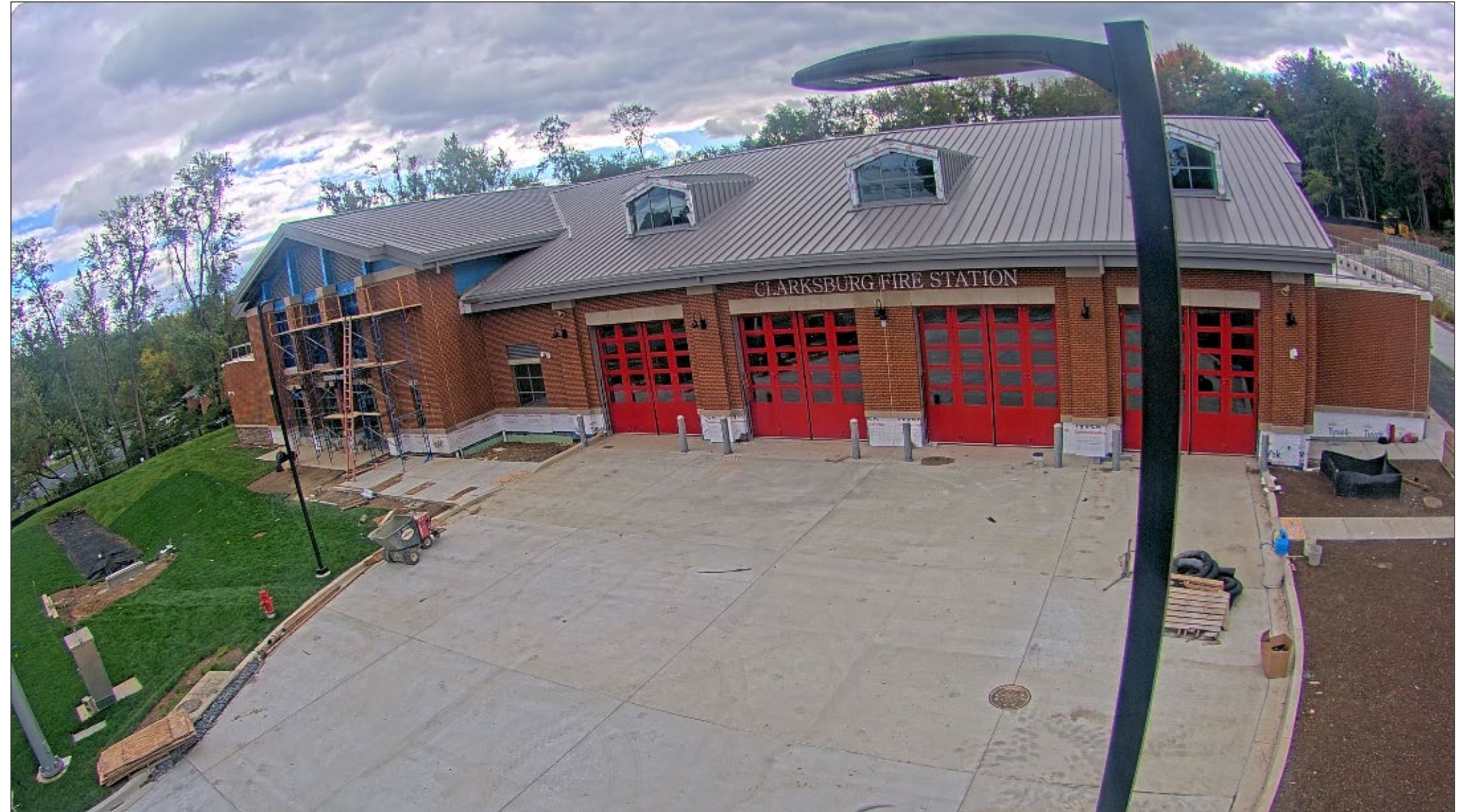
Construction progress as of October 15, 2023. Image source: Montgomery County Department of General Services
