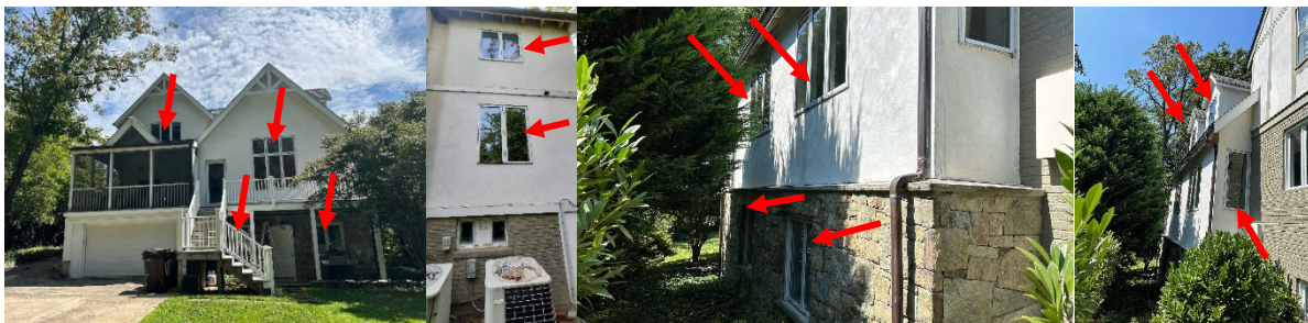
Figure 3: View of the rear and side elevations of the ca. 1997 addition, 2023. The red arrows point to the windows to be replaced. Source: Montgomery Planning.
