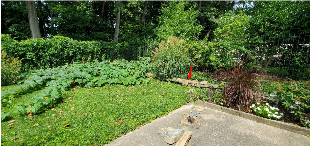
Figure 4: View of the existing stone retaining wall, 2023. Source: Montgomery Planning.
