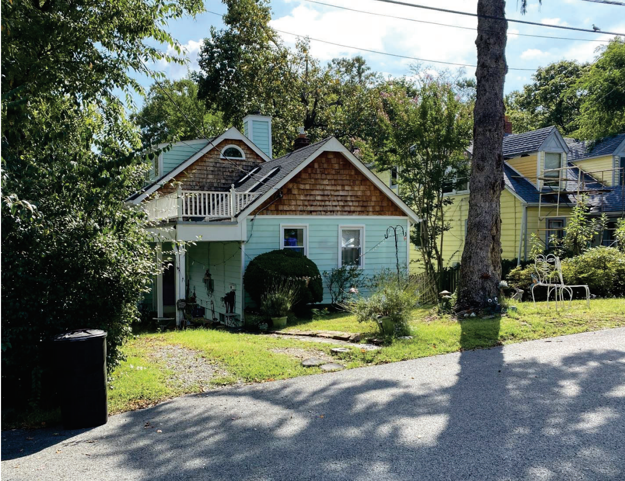
Figure 3: Replacement sash and half-round windows installed, 2023.
