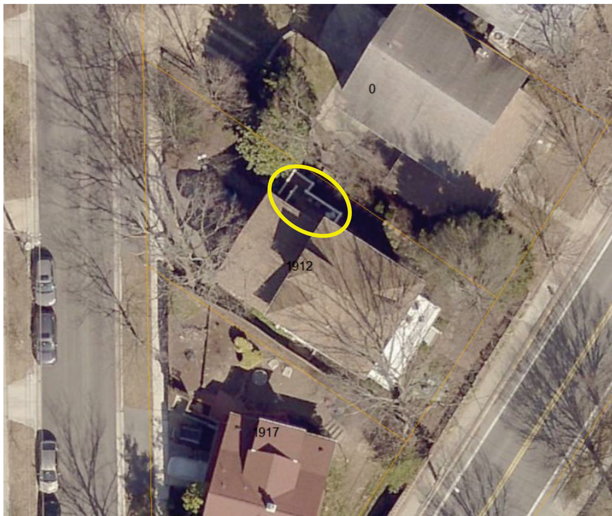
Figure 2: Aerial photo of the subject property with the deck circled in yellow.
