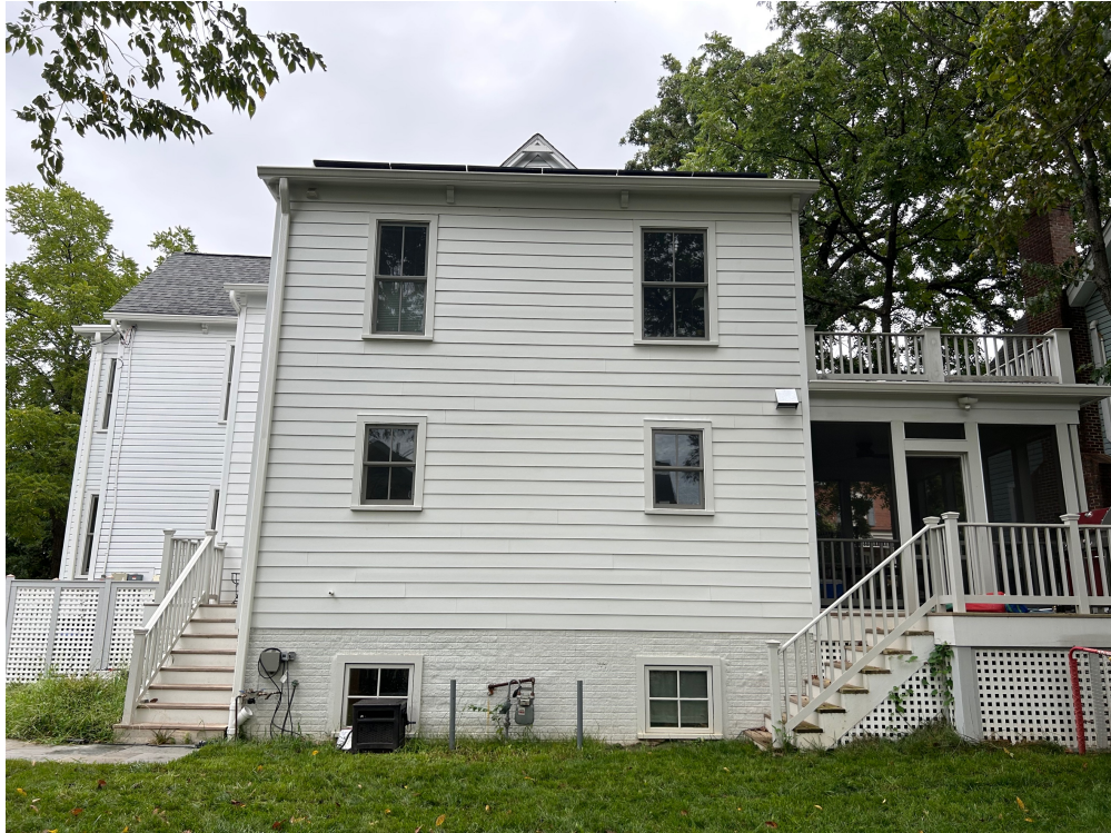
SOUTH ELEVATION – FACING 8 PINE AVENUE
