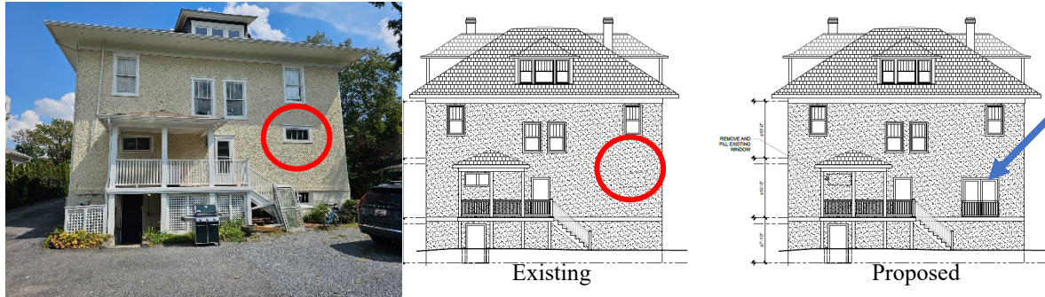
Figure 4: View of the rear elevation of 6812 Connecticut Avenue (left), the existing rear elevation as shown in the application (middle), and the proposed rear elevation (right) as shown in the application. Please note the missing four-light window (circled red) on the existing elevation and the proposed French doors (blue arrow).
