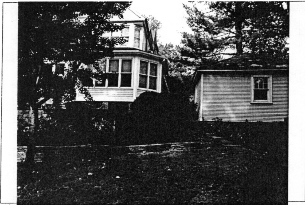
Detail: This photo was taken standing close to the rear property line, looking toward the rear facade of the house/garage.
