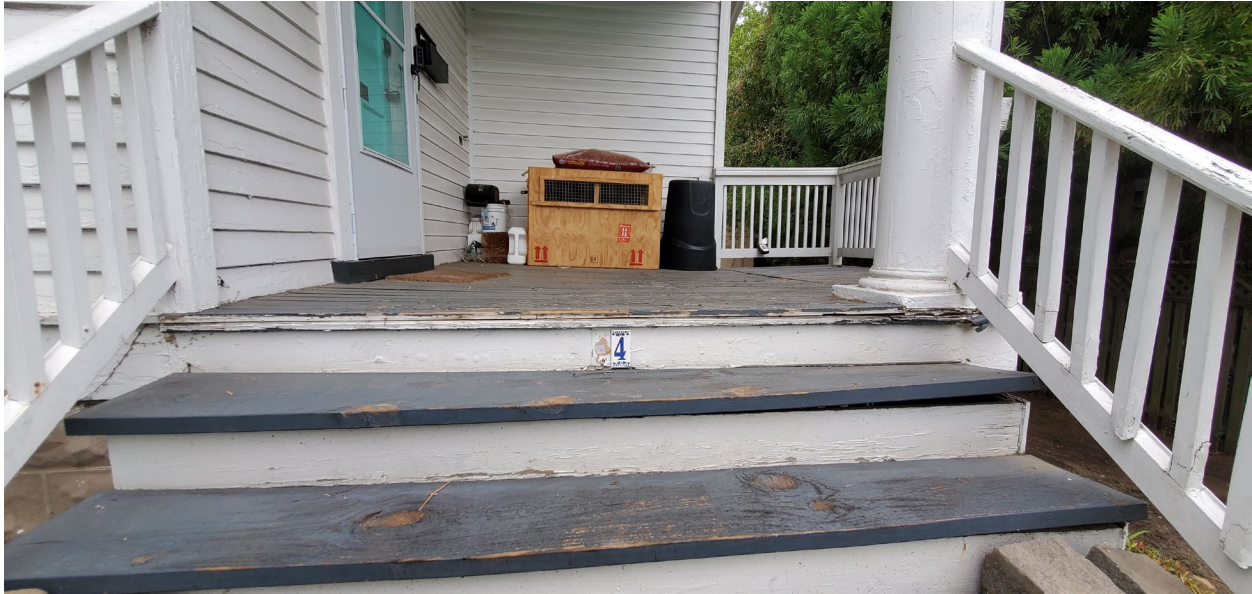
Figure 5: View of the front porch flooring. Source: Montgomery Planning.
