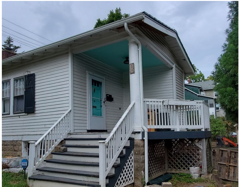
Figure 4: View of the porch addition to be demolished. Source: Montgomery Planning.
