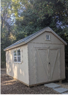
Figure 10: View of the installed shed.
