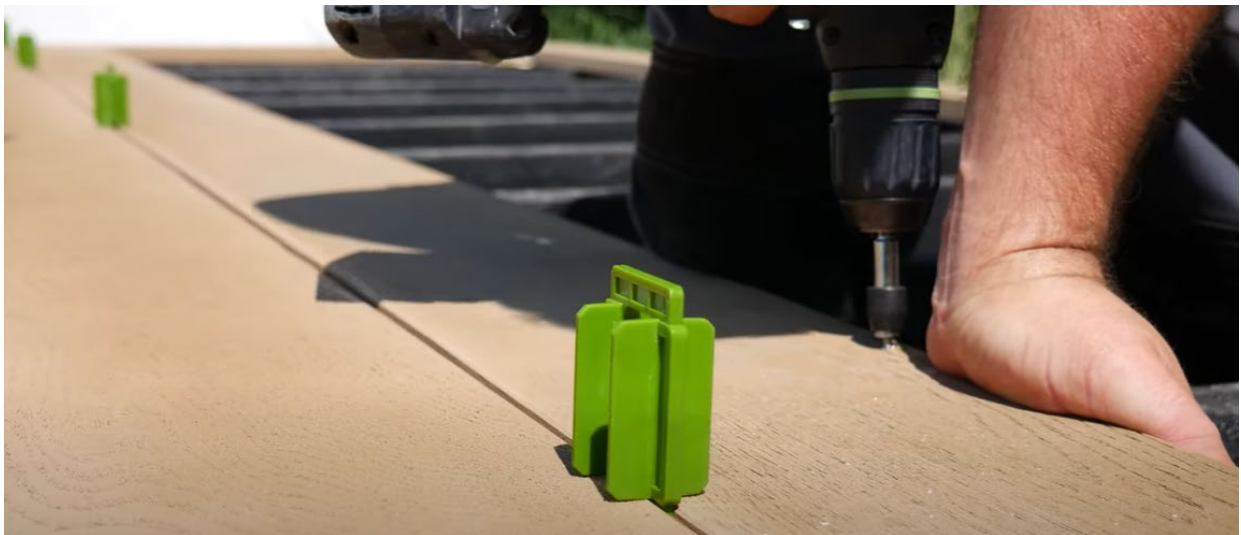
Figure 7: Example of Millboard installation. Source: Millboard (via Youtube).
