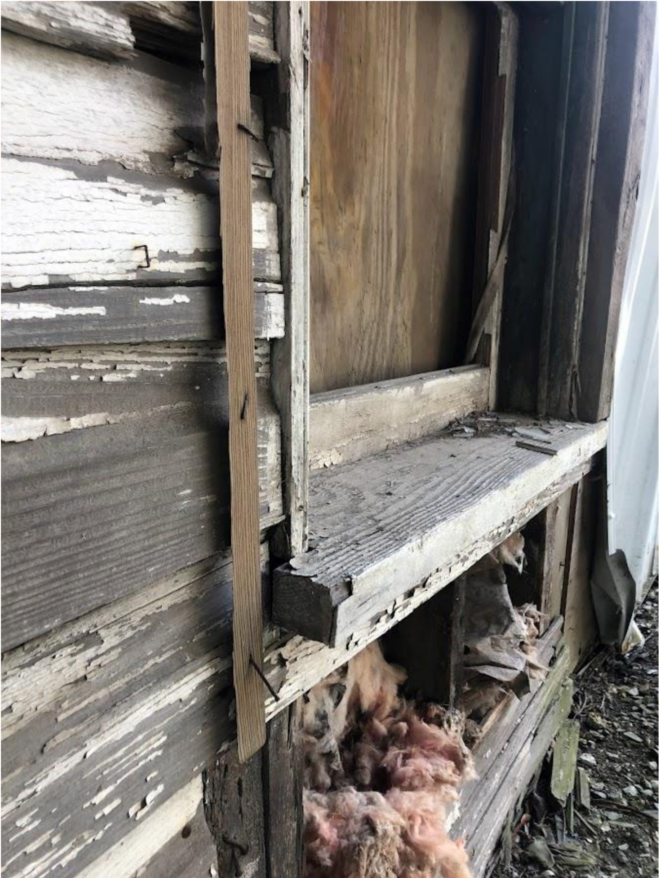
27. White Barn, First floor window sill detail. Photo number 7288.
