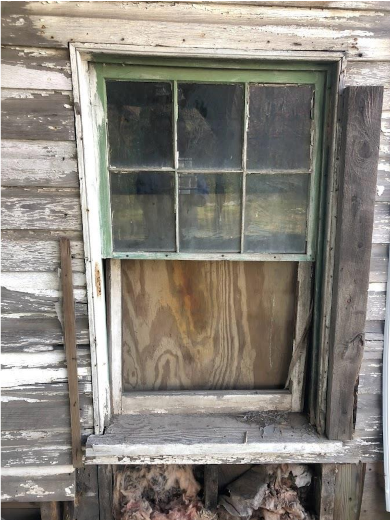
24. White Barn, First floor window detail on north elevation. Photo number 7170.
