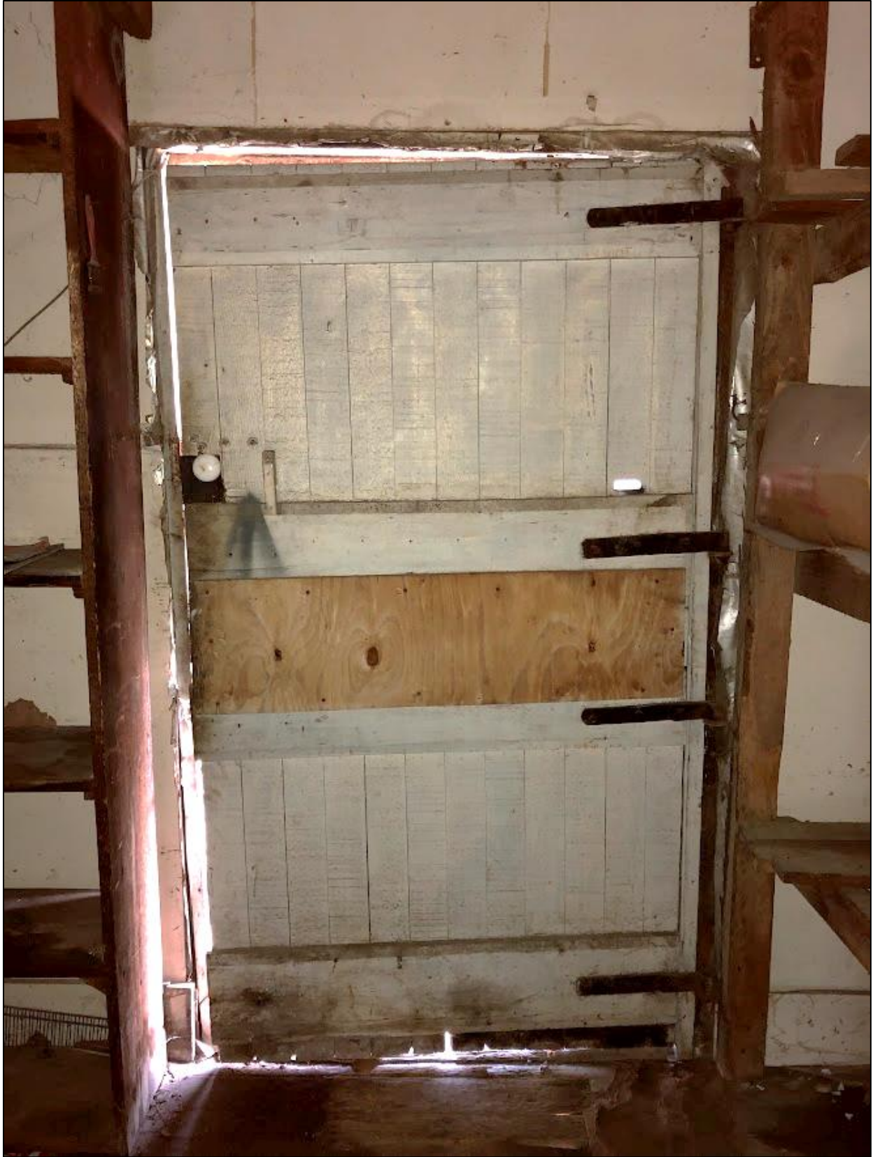
6. Smith Hoyle's Mill, Interior view of front door.
