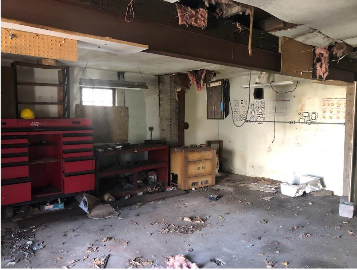
33. White Barn, West room, north and east walls. Photo number 7255.
