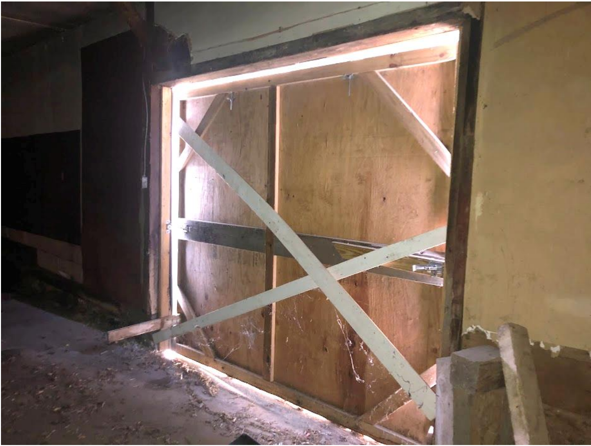
45. White Barn, East room, south door detail. Photo number 7270.
