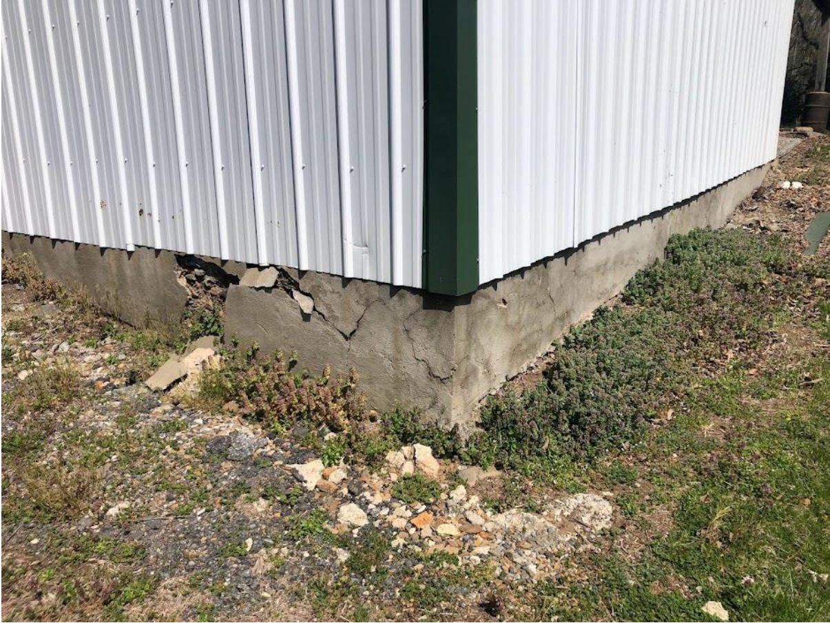
22. White Barn, View northwest at southeast foundation corner. Photo number 7298.
