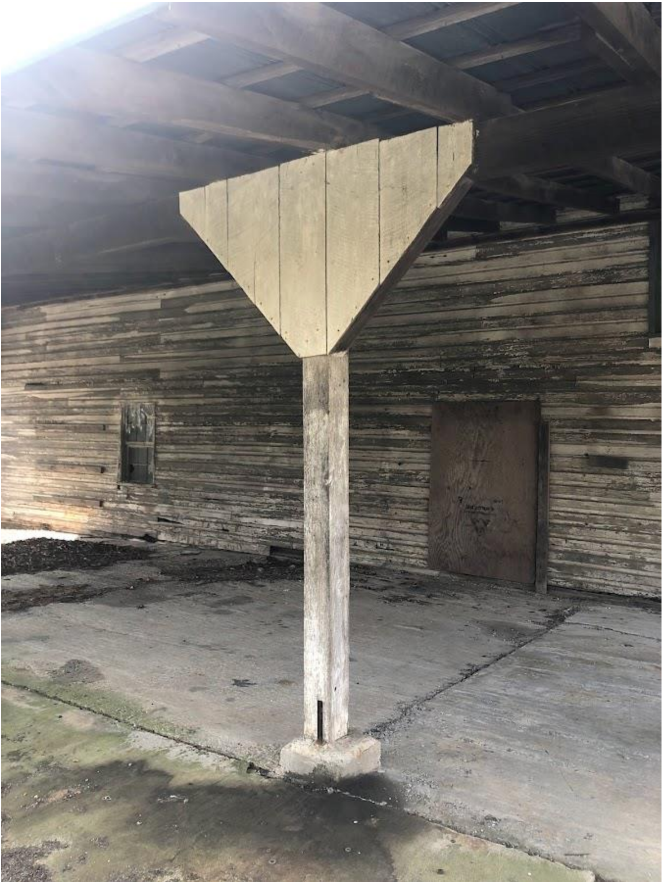
15. White Barn, North truck port center support post exterior. Photo number 7169.
