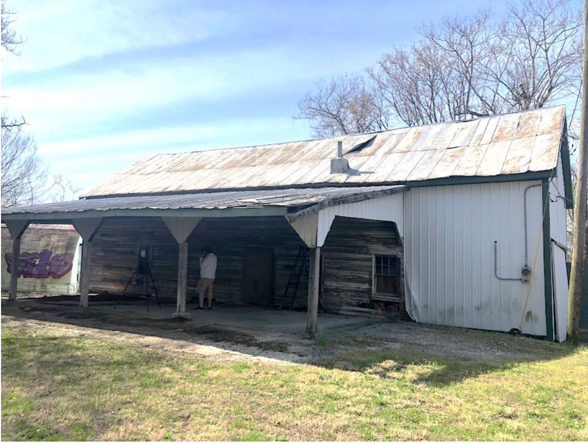
4. White Barn, North elevation and truck port shed addition. Photo number 7253.
