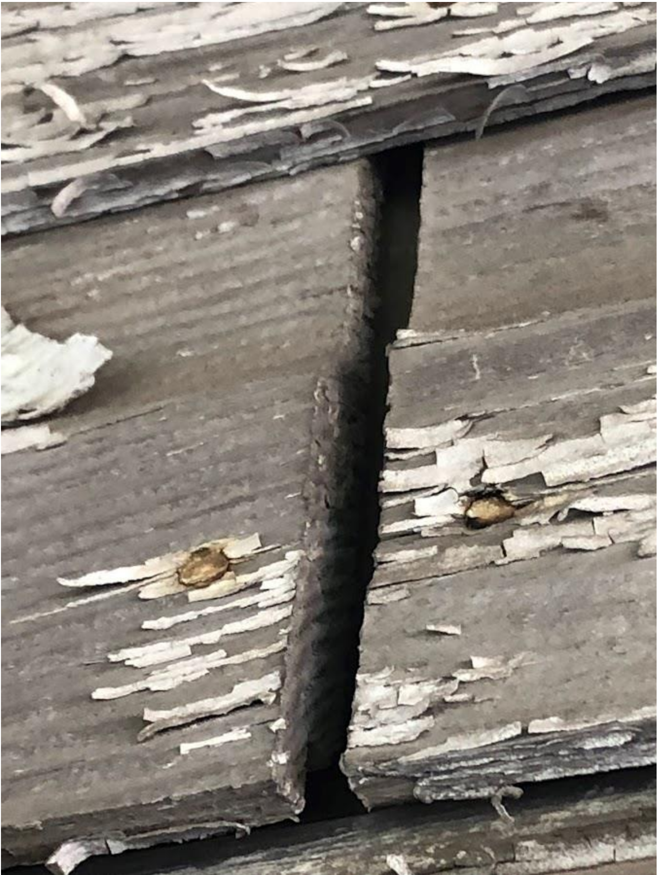
30. White Barn, Dutch lap siding detail, north elevation. Photo number 7180.
