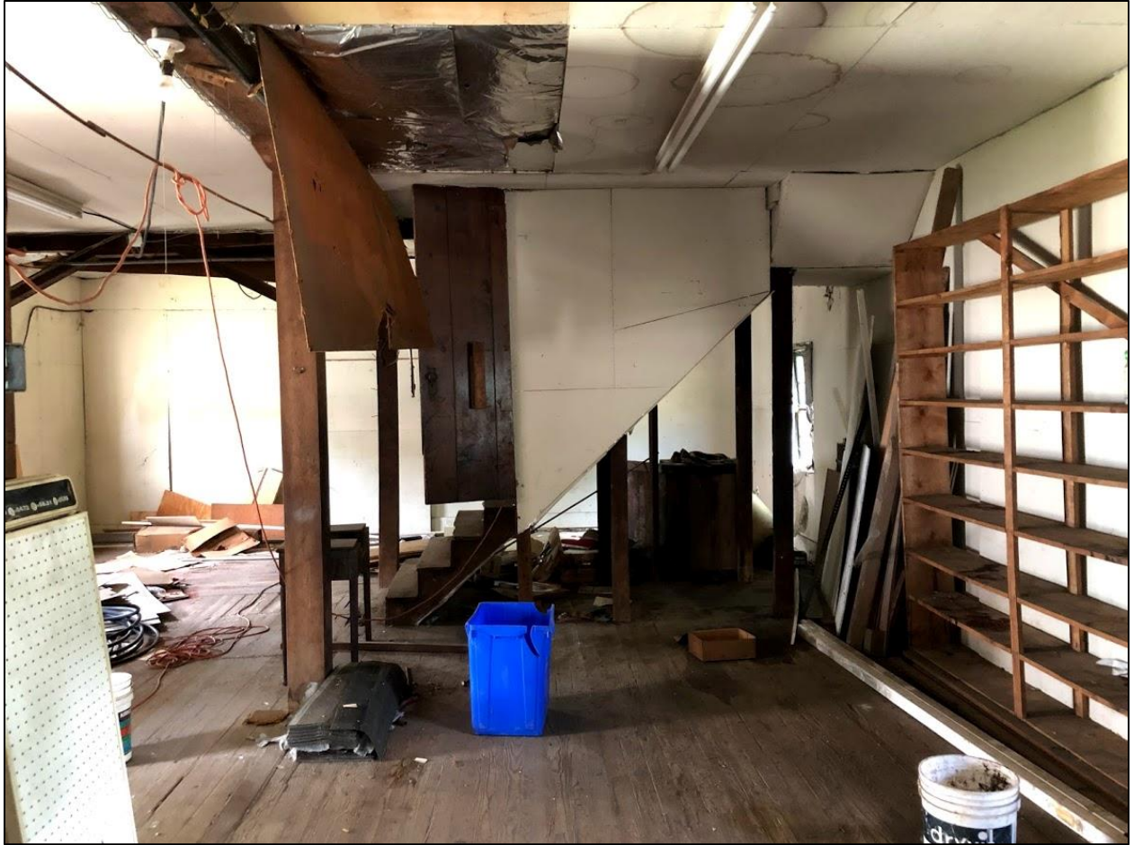
9. Smith Hoyle's Mill, Interior view east towards stairs to second floor.
