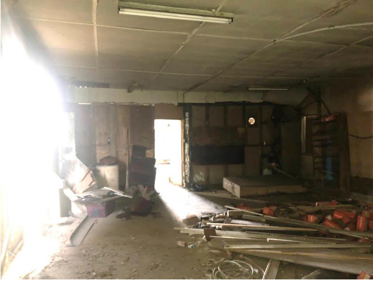
46. White Barn, East room, west wall. Photo number 7271.
