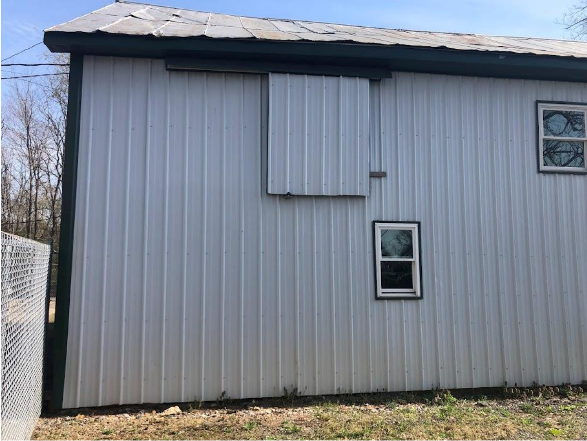
10. White Barn, South elevation, west half. Photo number 7228.
