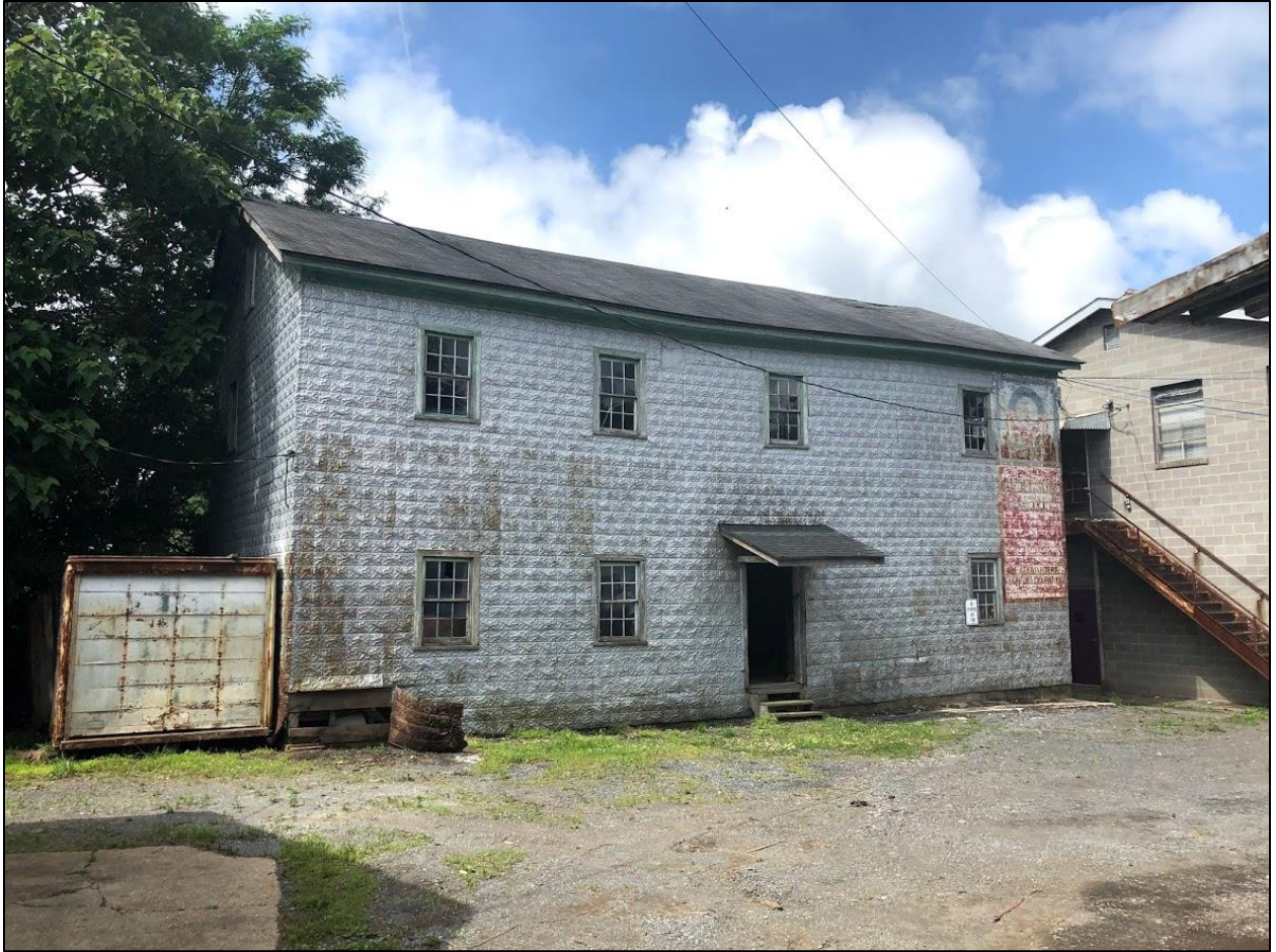
1. Smith Hoyle's Mill, North elevation.
