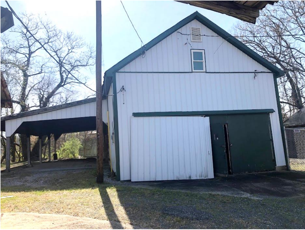
2. White Barn, West elevation. Photo number 7155.
