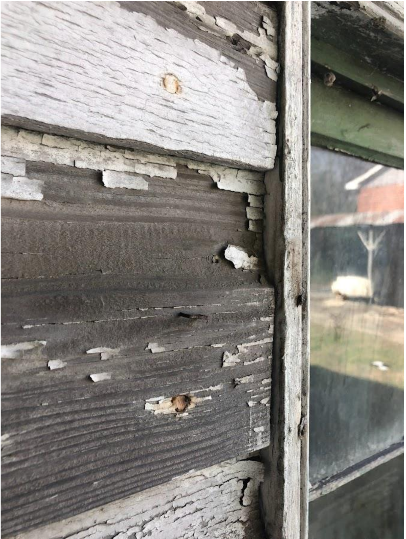
29. White Barn, Dutch lap siding detail, north elevation. Photo number 7179.
