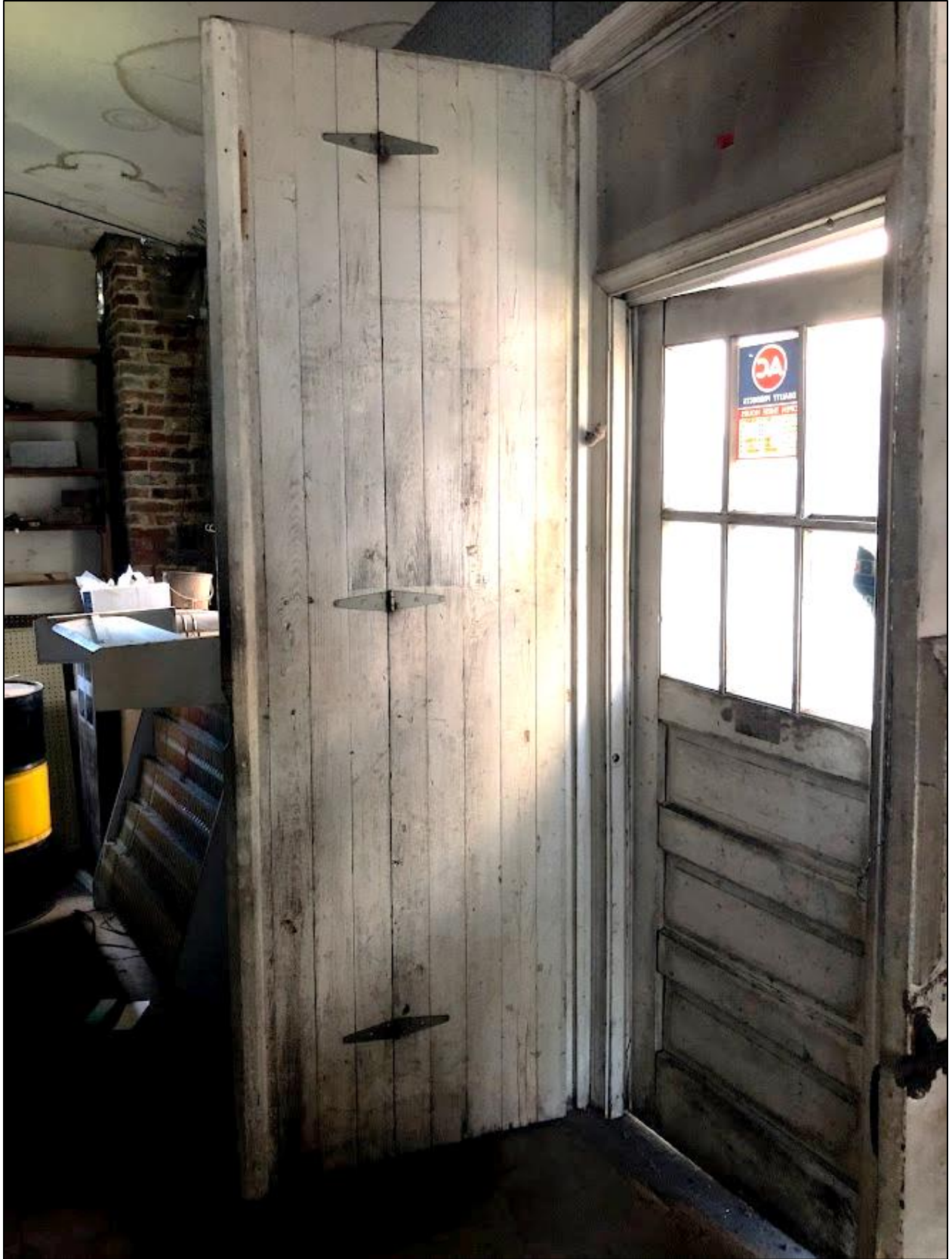
8. Smith Hoyle's Mill, Interior view of west bi-fold inner door opened revealing outer door of later date.
