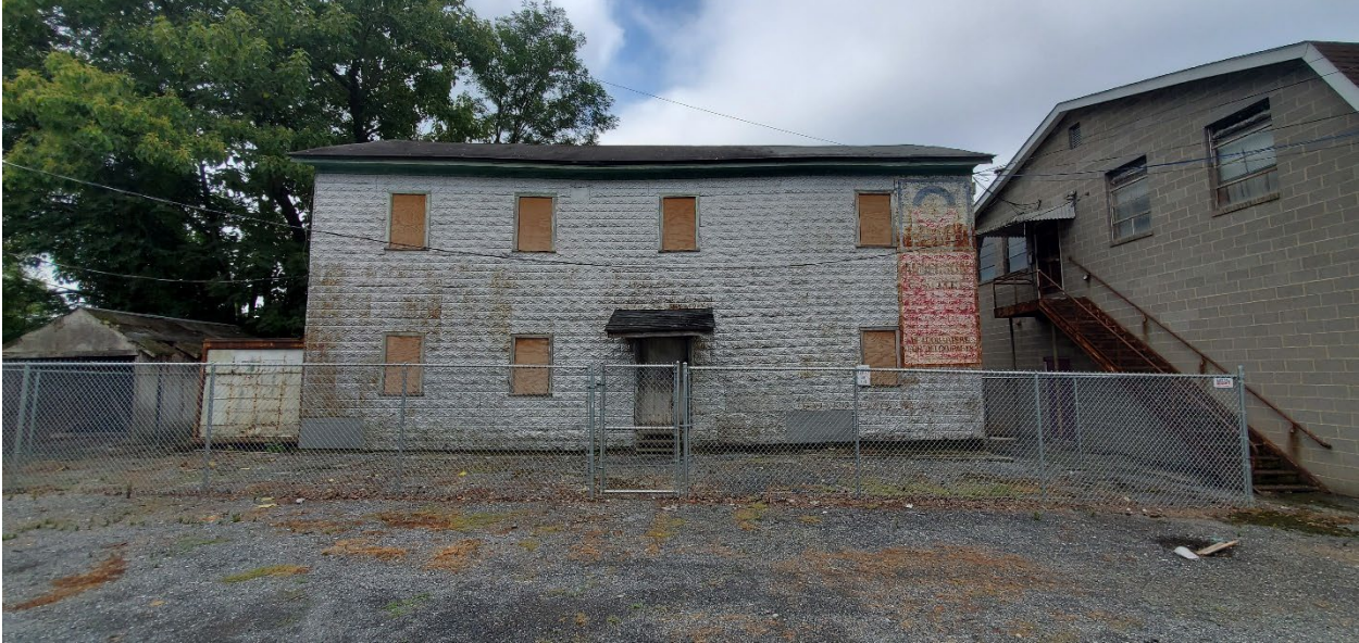
Figure 7: View of the facade of Hoyle's Mill, 2023.
