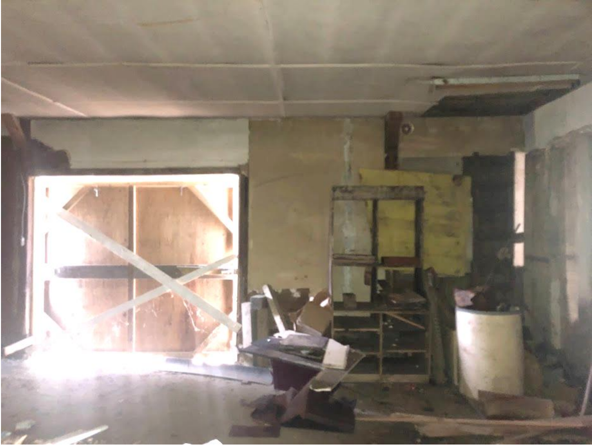
44. White Barn, East room, south wall. Photo number 7275.
