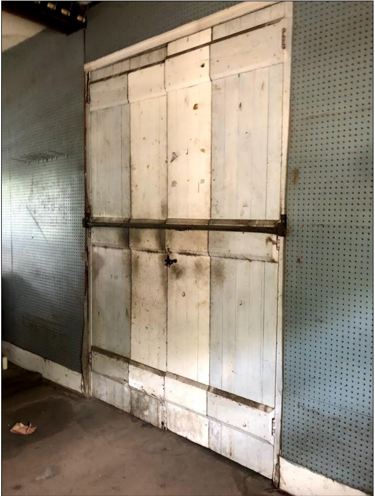
7. Smith Hoyle's Mill, Interior view of west door.
