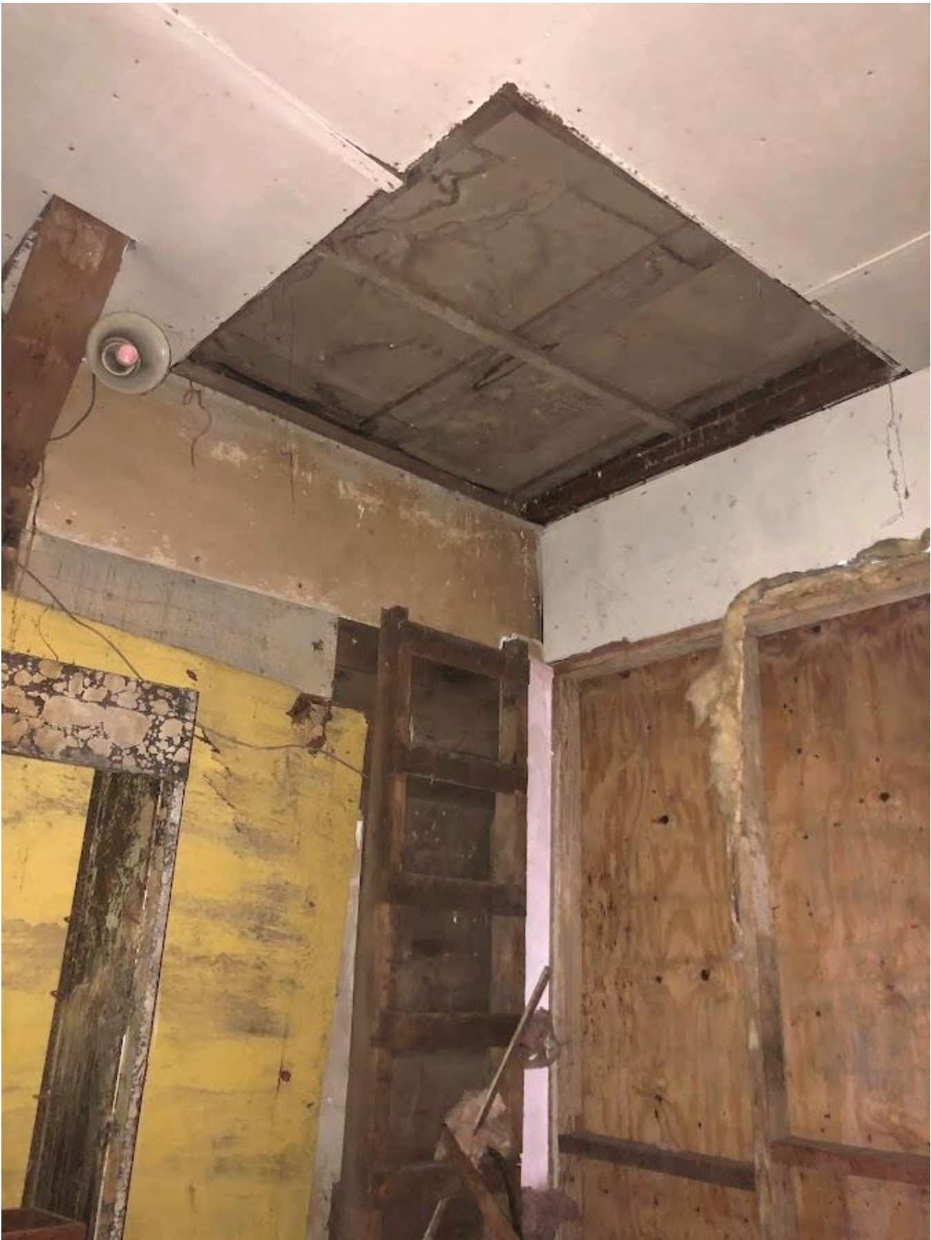
47. White Barn, East room, ladder to ceiling hatch detail. Photo number 7269.
