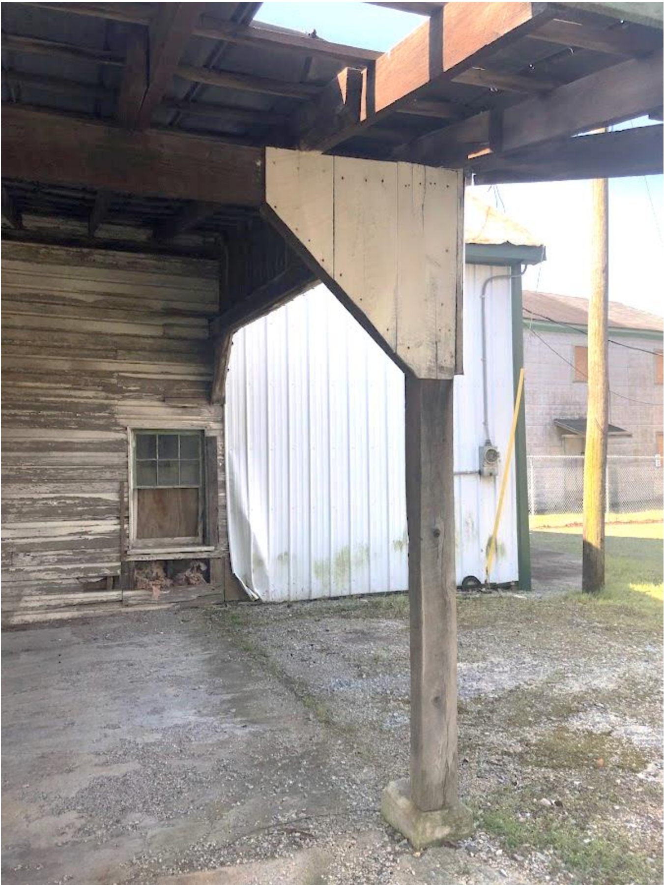
14. White Barn, Northwest truck port support post exterior. Photo number 7168.
