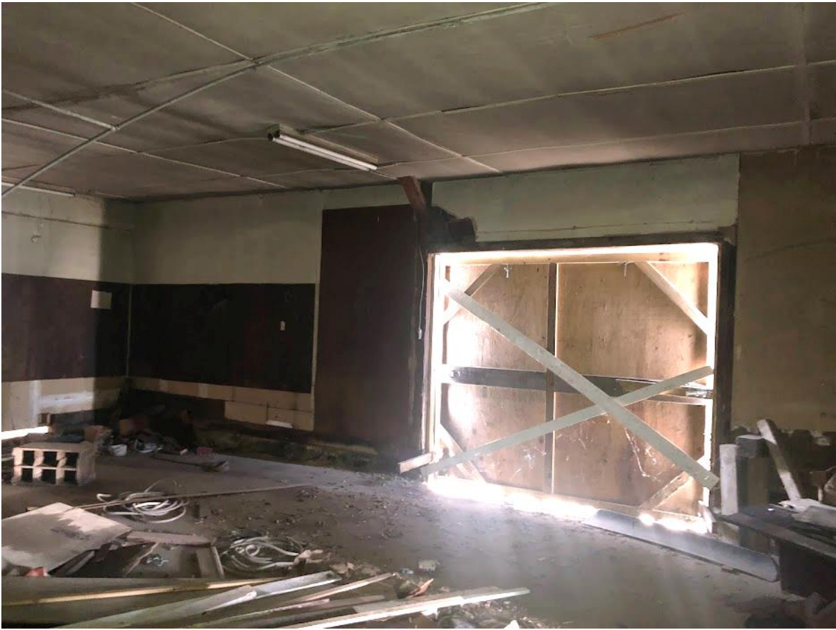
43. White Barn, East room, south wall. Photo number 7274.
