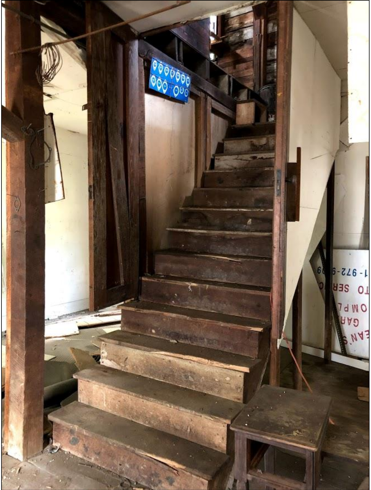
10. Smith Hoyle's Mill, Interior view of stairs to second floor.
