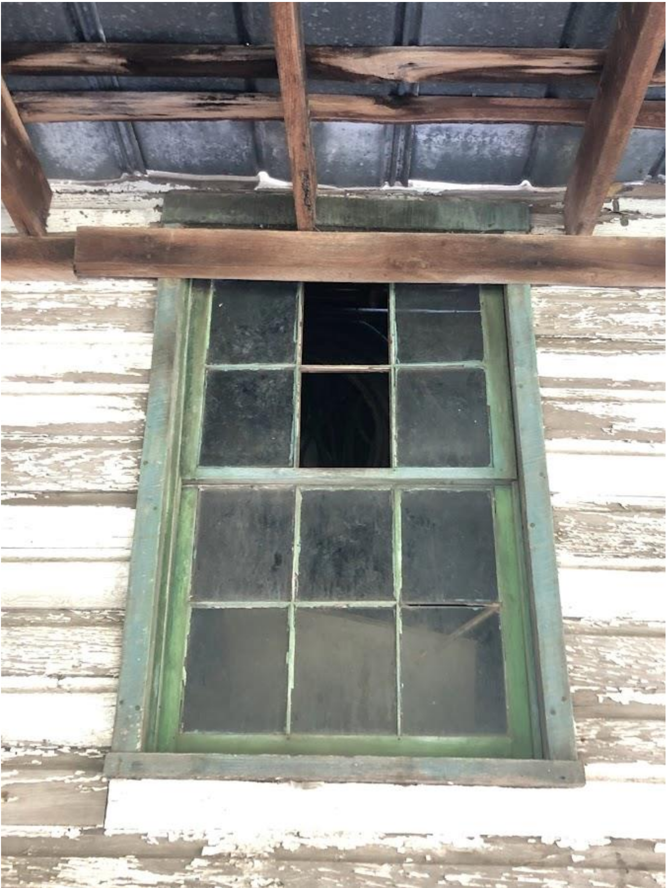
28. White Barn, Second floor window detail on north elevation. Photo number 7176.
