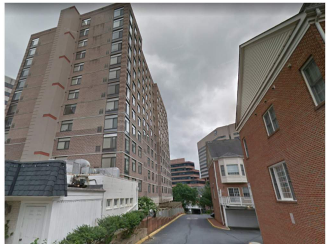
8 RAMSEY AVENUE LOOKING WEST
