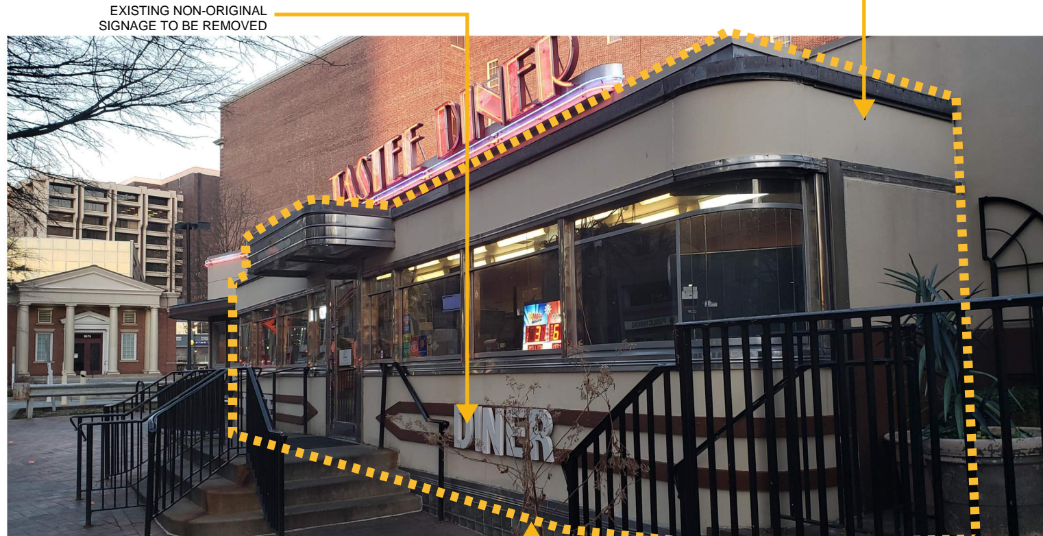
EXISTING VIEW FROM NORTHWEST
