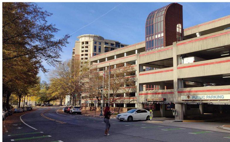
6 VIEW FROM CAMERON STREET LOOKING WEST
