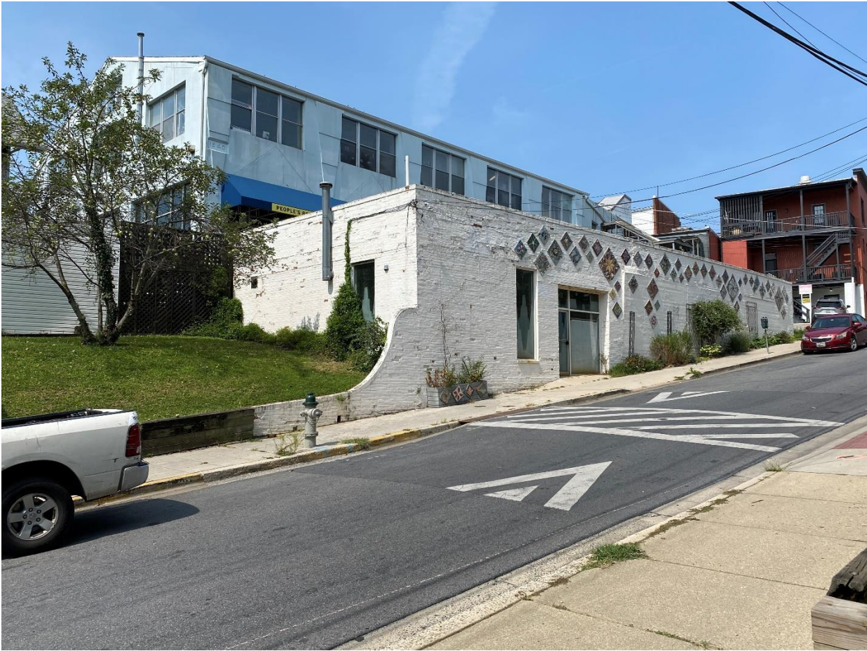
Figure 4: Current condition of the proposed patio location.
