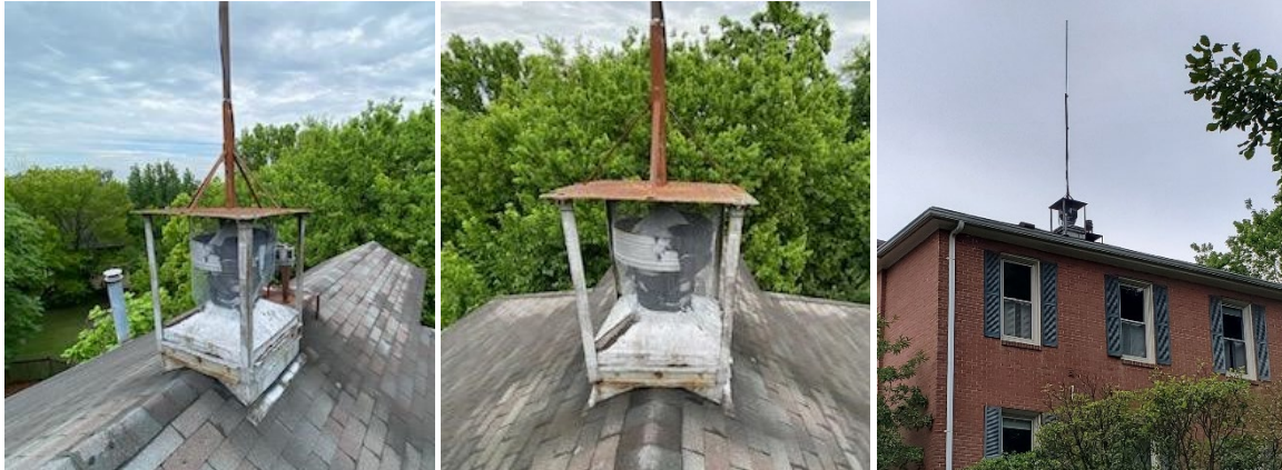
Figure 3: View of the antennae and associated equipment, 2022-2023. Source: Applicant and Google.
