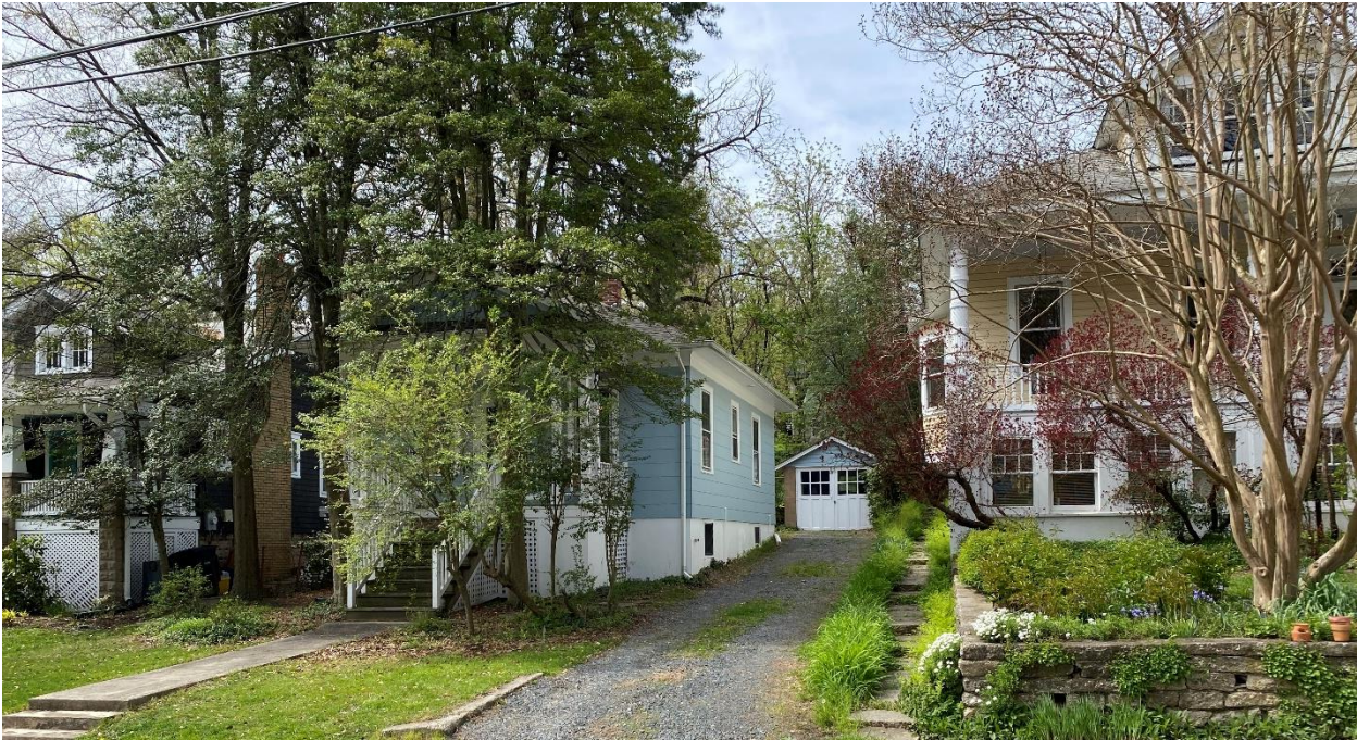
Figure 4: View along the right side of the subject property with the garage in the rear yard.
