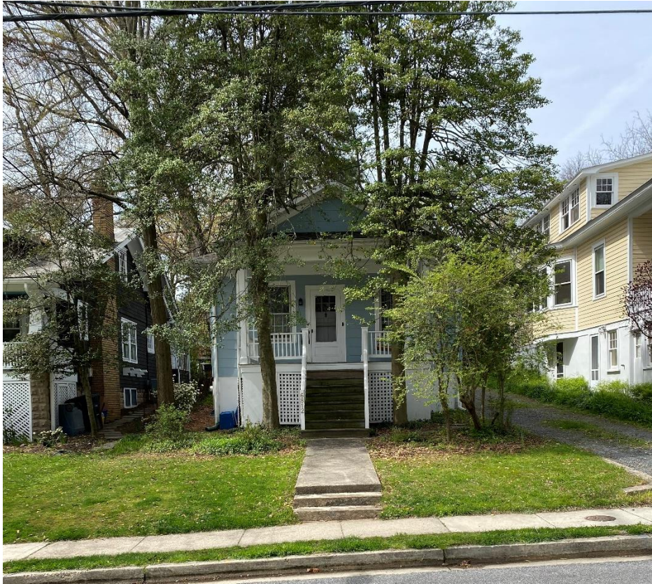
Figure 2: Front elevation of the subject property.
